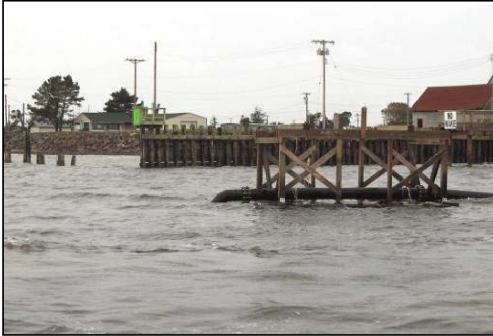
Figure 8. Anchored dredge discharge diffuser float for flowlane disposal 5 ft below water surface.
