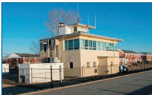
Combatant Craft Division Waterfront Operations Facility, Ft Monroe. U.S. Navy Photo.
