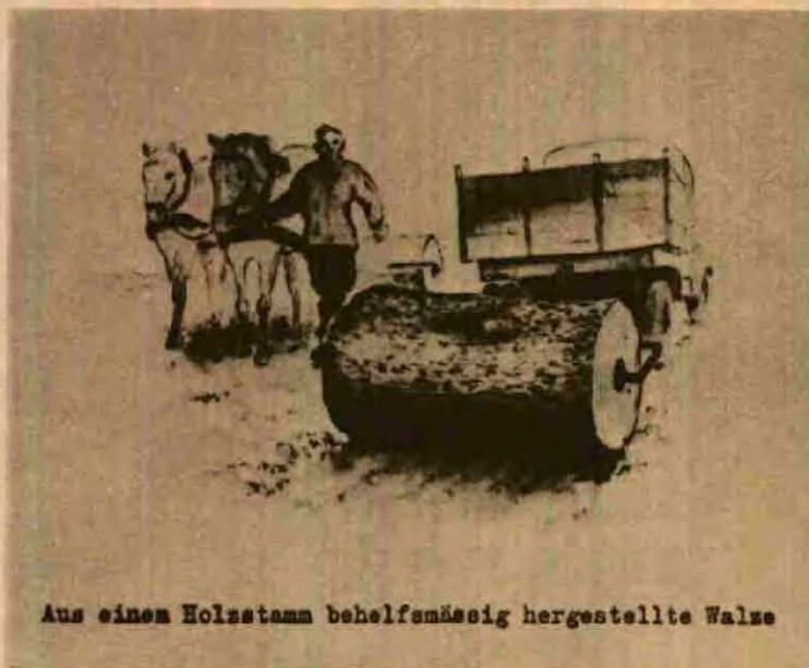
(An Emergency Roller Made From a Tree-trunk)
