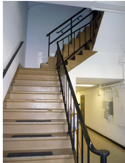
Modular Stairs over Existing Stairway at Naval Base San Diego, CA
