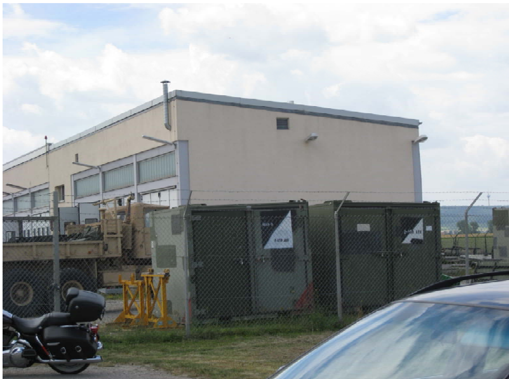
Figure 72. Motor Pool Bldg 6633 – Illesheim.
