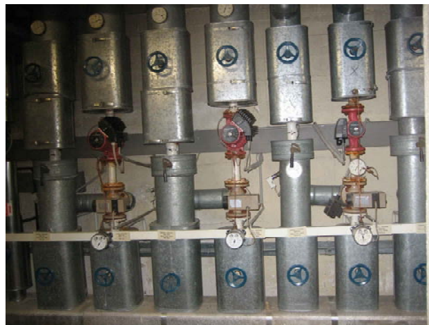
Figure 99. Example heating circulation pumps.
