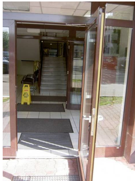
Figure 30. Bldg 18 front door propped open.
