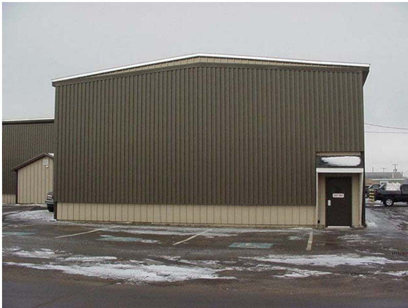
Figure 86. Building with solar wall.
