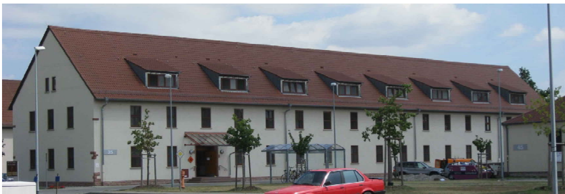
Figure 50. Bldg 35/Barracks – Mannheim.
