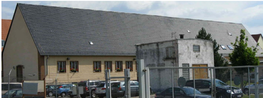
Figure 67. Bldg 5819/Office – Ansbach.
