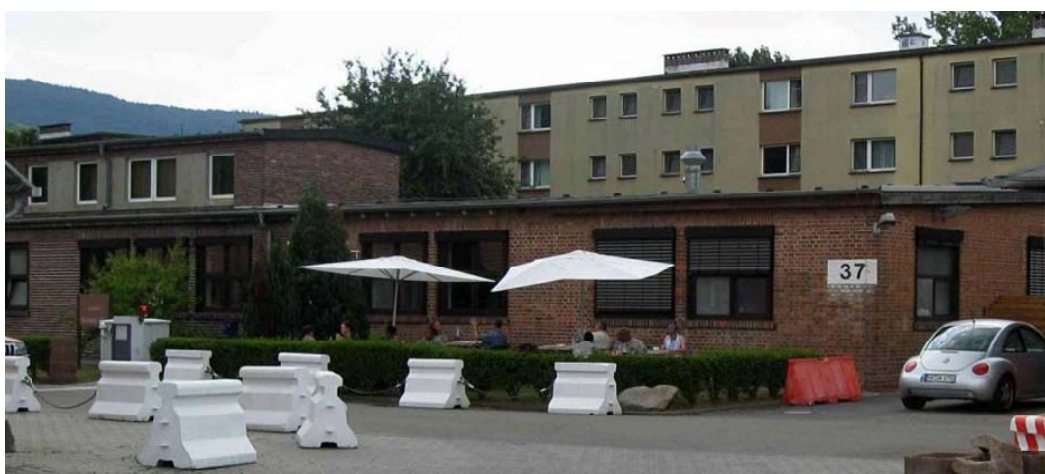
Figure A11. Bldg 37/Dining Facilities at Heidelberg.
