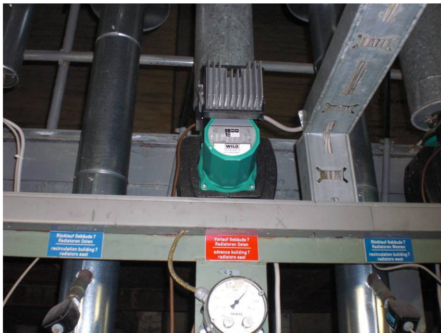
Figure 27. Wilo-P analog pump.
