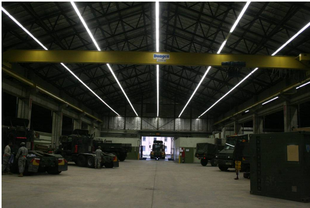
Figure 46. Maintenance area with no skylights.
