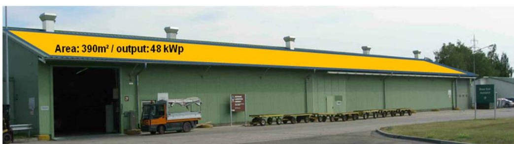
Figure 24. Example PV-system – Bldg 7889 Germersheim.
