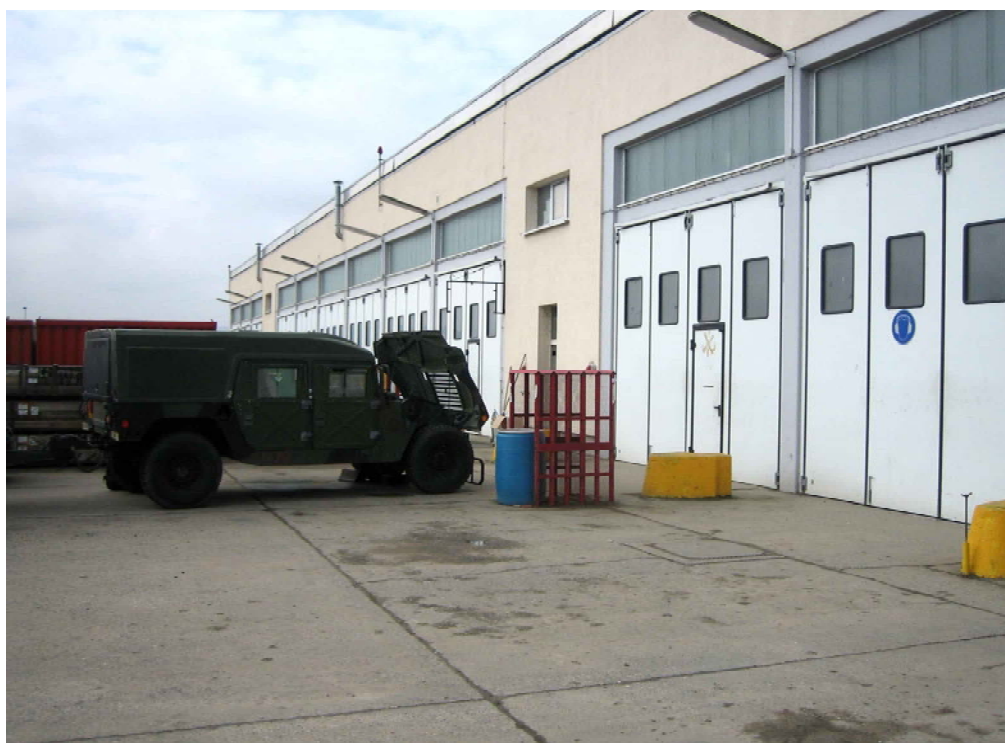
Figure 61. Bldg 6633 – Motor Pool 1.
