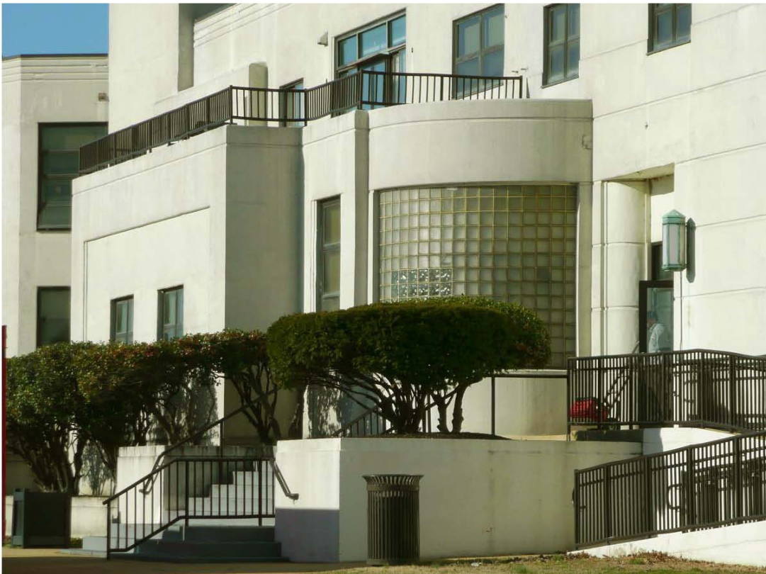
Building 92 – close-up of entry and original curved glass block wall on the east elevation
