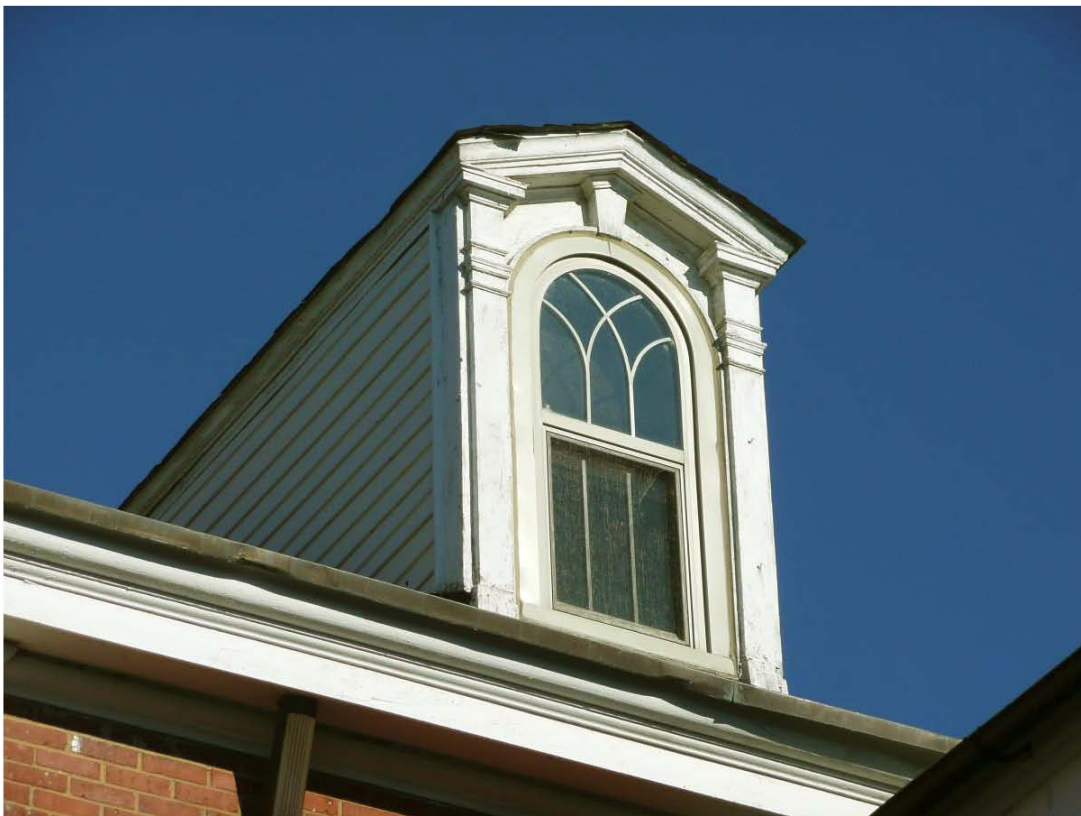
Building 72 – attic dormer on gymnasium addition
