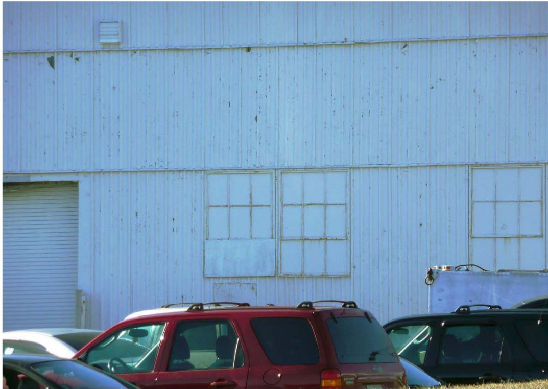
Building 97 – windows on the north elevation
