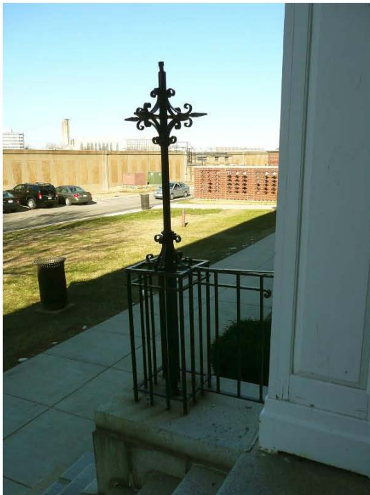
Building 72 – original wrought iron railing and light fixture on west elevation
