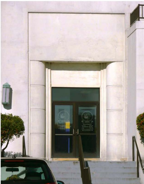
Building 92 – door detail on east elevation
