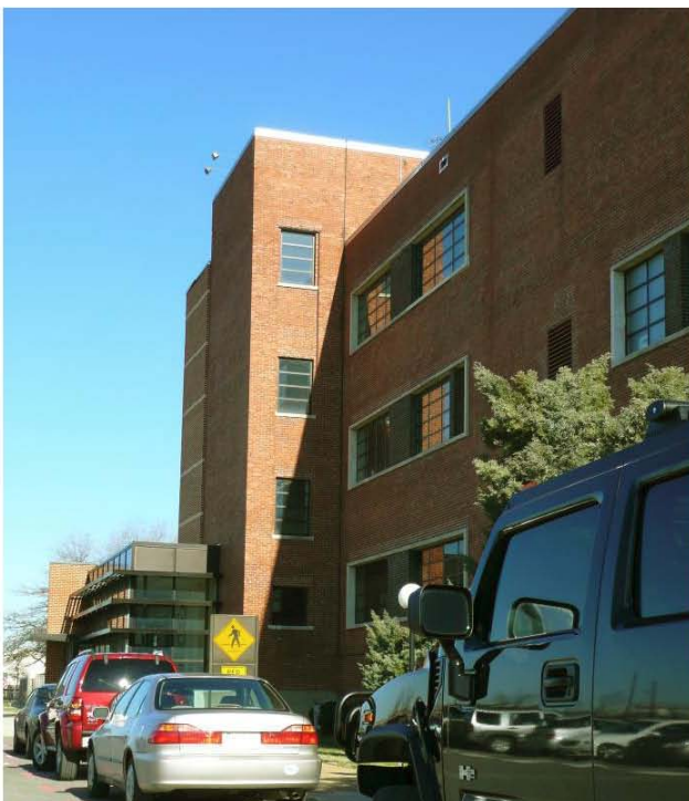
Building 168 – stairwell detail on west elevation
