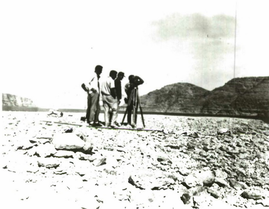
Figure 8.--View of transitman directing boat on a given azimuth.
