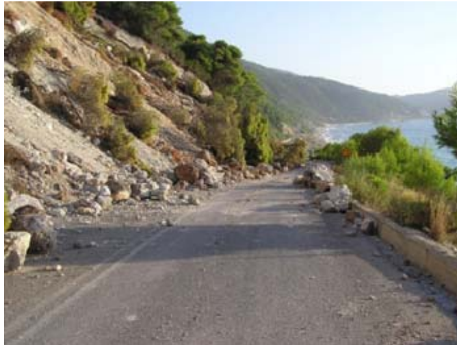
Figure 17. Landslide in Pefkoulia on Lefkada Island (next to Kefalonia in the Ionian Sea), after the 2003 M 6.4 earthquake (From: Papadopoulos, Karastathis, Ganas, Pavlides, Fokaefs, & Orfanogiannaki, 2003)
