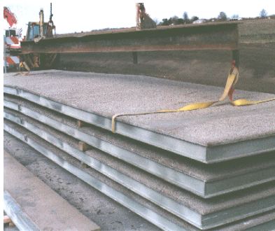
Figure 5. FRP composite bridge deck panels for installation on Kansas State Highway 126 west of Pittsburg, Kansas. Panels manufactured by Kansas Structural Composites Inc.
