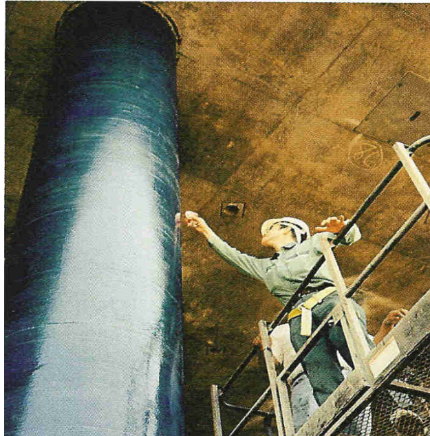
Figure 10. MBrace CFRP composite from Master Builders Technologies being applied to a concrete bridge column.
