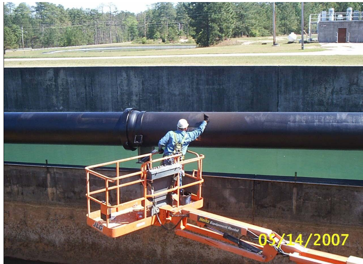
Figure 21. Applying smart coating system to pipe.
