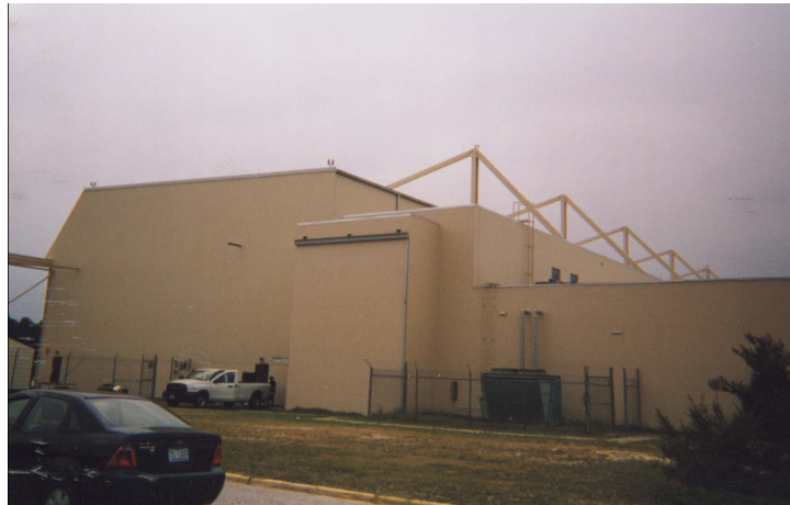
Figure 4. Simmons AAF hangar after overcoating has been completed.
