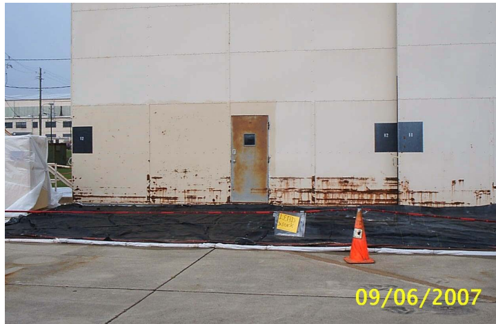
Figure 9. Simmons AAF hangar before painting.
