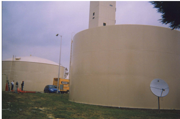
Figure 3. Deluge tanks after overcoating.
