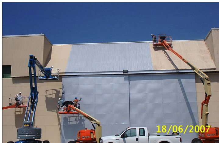
Figure 13. Simmons AAF hangar during overcoating.
