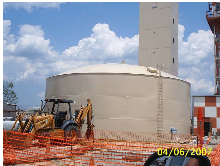
Figure 36. Deluge tank with newly completed overcoat system.
