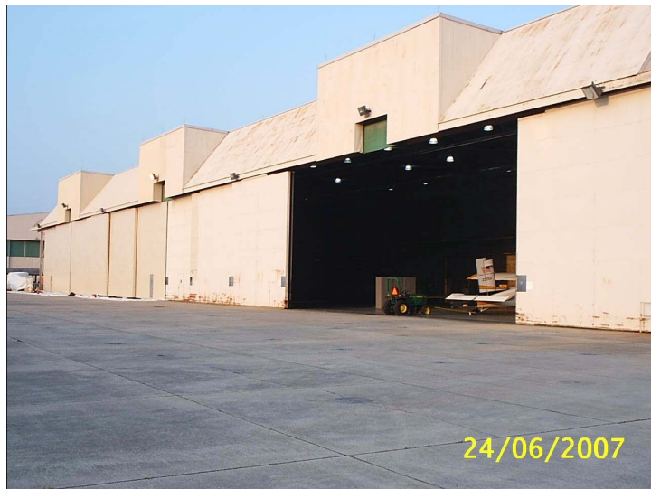
Figure 7. Simmons AAF hangar before painting.
