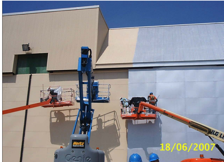
Figure 12. Simmons AAF hangar during overcoating.
