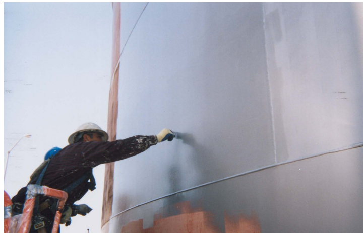
Figure 18. Inspecting the paint thickness on a deluge tank.
