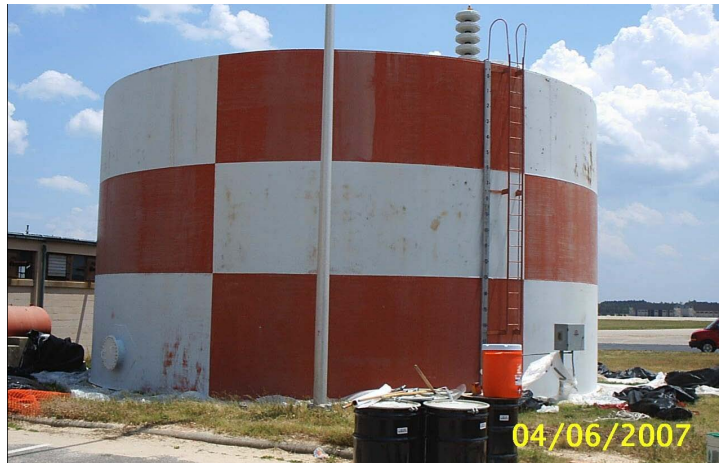
Figure 30. Deluge Tank No. 1 before painting.
