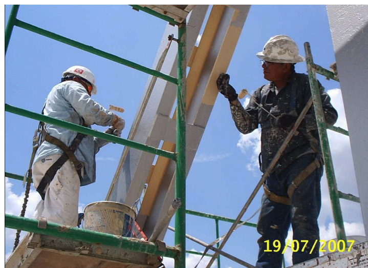
Figure 29. Painting the hangar superstructure.
