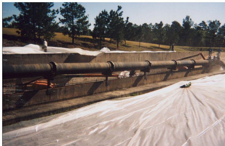
Figure 20. Before applying smart coatings (note ground tarps for environmental protection).
