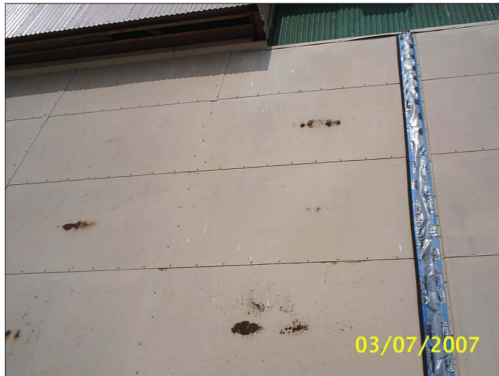
Figure 10. Simmons AAF hangar before painting, showing masking of utility line.
