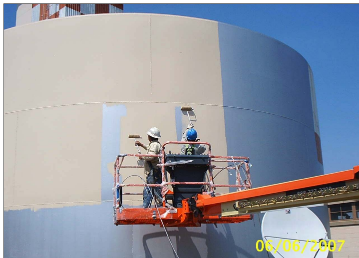
Figure 31. Applying aliphatic polyurethane topcoat to deluge tank.
