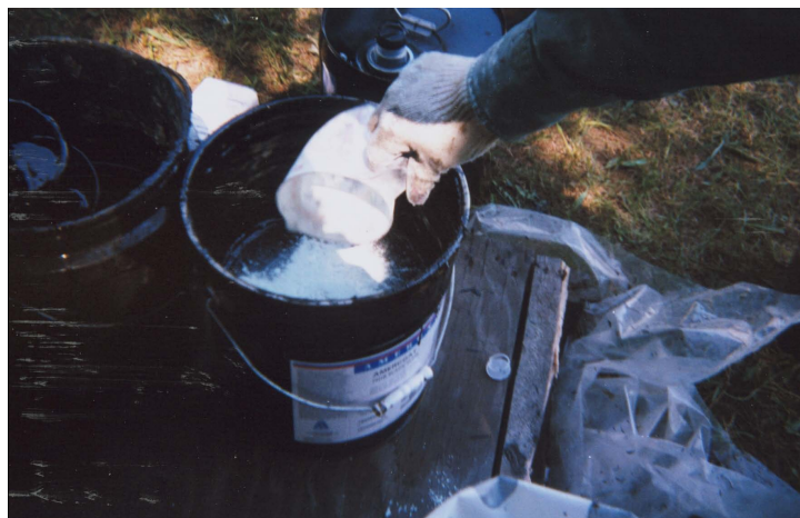
Figure 26. Mixing the coal tar epoxy with UVITEX OB fluorescent pigment.
