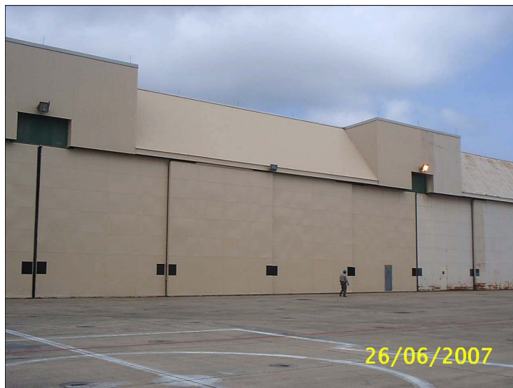
Figure 5. Simmons AAF hangar work in progress.
