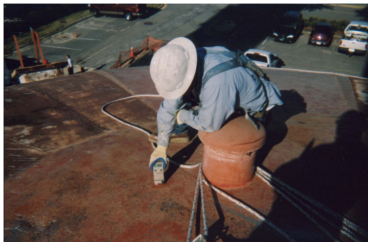
Figure 35. Inspecting the deluge tank paint thickness before starting work.
