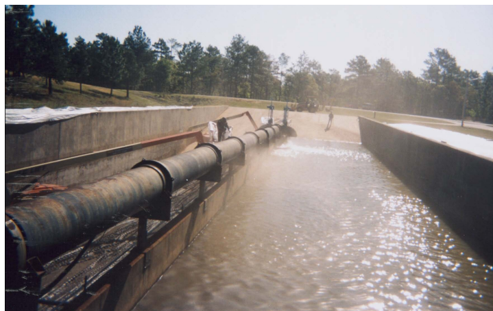
Figure 22. Abrasive blasting the pipe before applying smart coatings.
