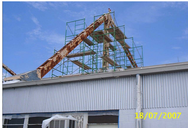
Figure 27. Scaffolding in preparation for work on hangar superstructure.
