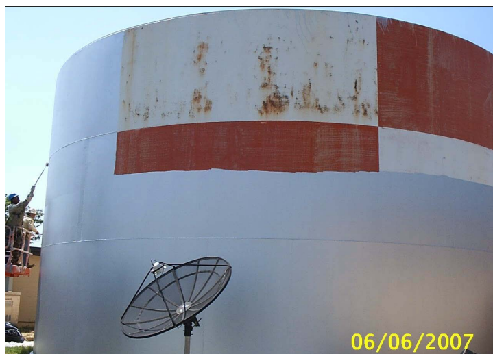
Figure 32. Work in progress showing the overcoat primer, an MCU (Rust Grip).
