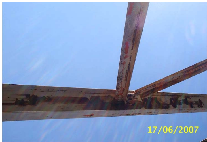
Figure 17. Simmons AAF hangar superstructure after power washing.
