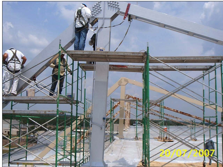
Figure 1. Overcoating the hanger superstructure (working from scaffolding and appropriately tied off).
