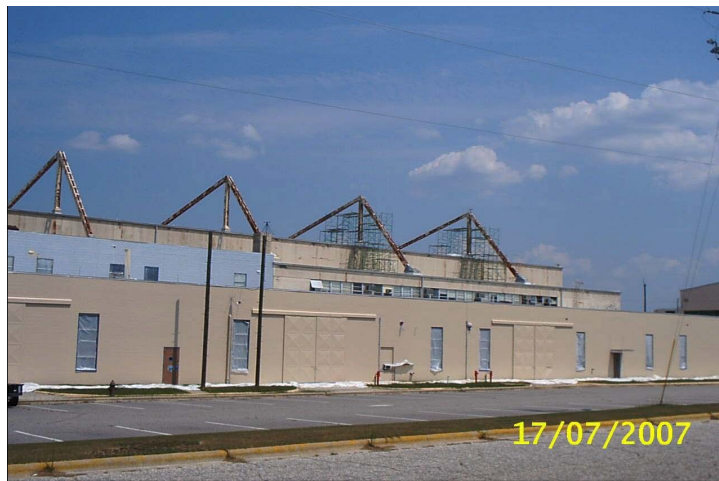
Figure 16. Simmons AAF hangar during overcoating.
