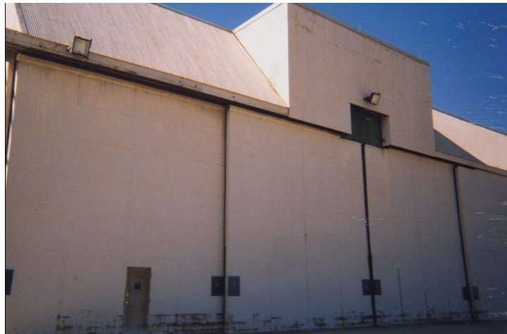
Figure 6. Simmons AAF hangar before painting.
