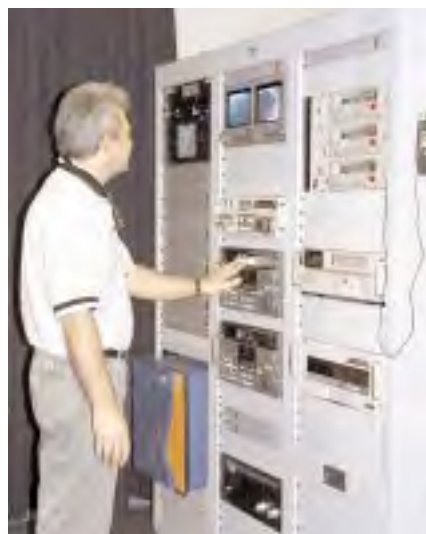
Above: The main rack contains six video sources, a dubbing station, routing hardware, and the base station for one of the nonlinear editors. The studio can accommodate eight different videotape formats and a variety of digital files.
