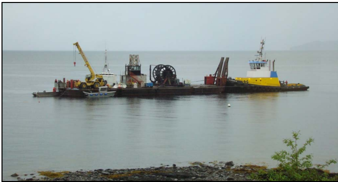
Figure 6 – Tugs and Cable Lay Barge during SEAFAC Cable Installation
