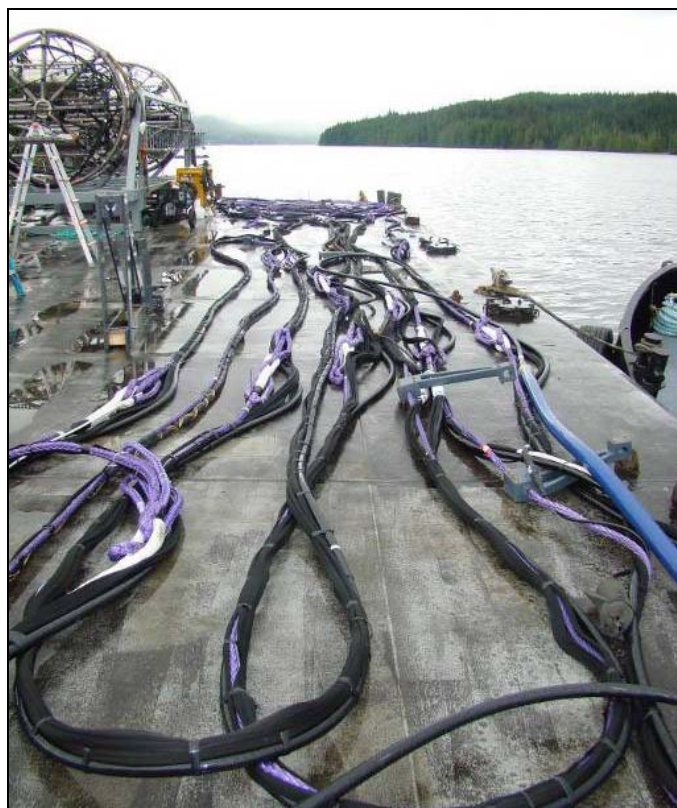
Figure 4 – Array Staging on Deployment Barge
