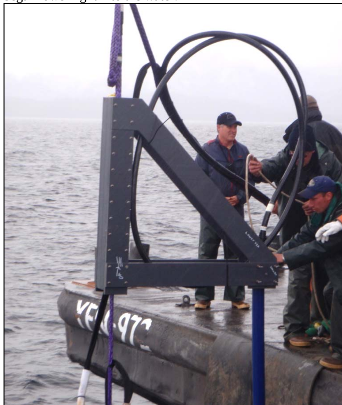
Figure 10 – Vector Sensor Array Installation
