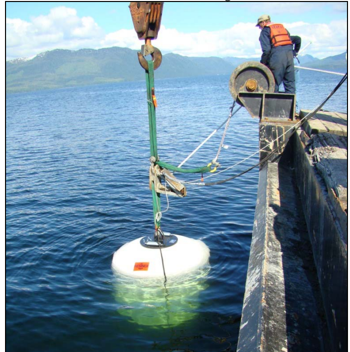
Figure 14 – Buoy Installation with Hydraulic Release
