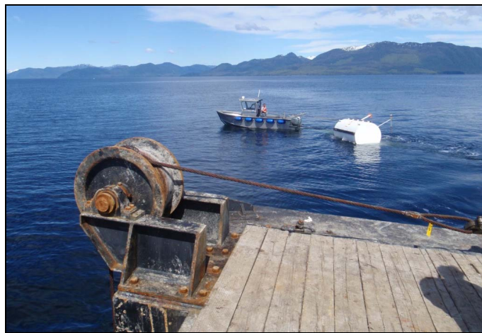
Figure 5 – Mooring Barge Mooring Buoy Installation
