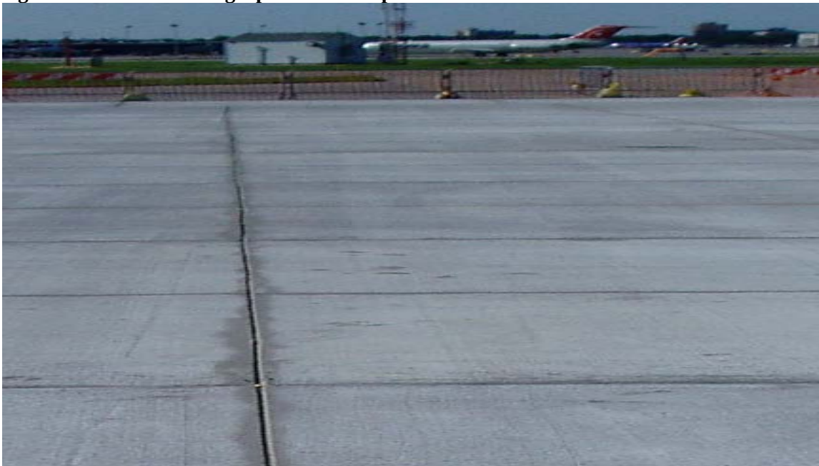
Figure 3. Aircraft Parking Apron After Repairs
