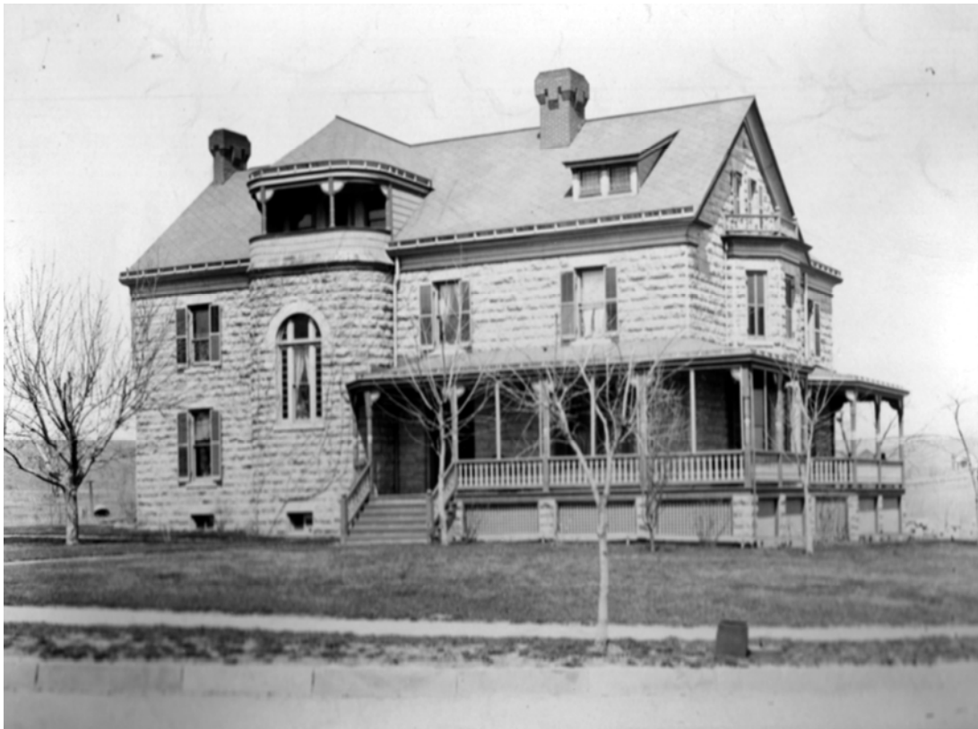
Figure 6. Commandant's Quarters, Bldg 1, circa 1900 (NARA).
