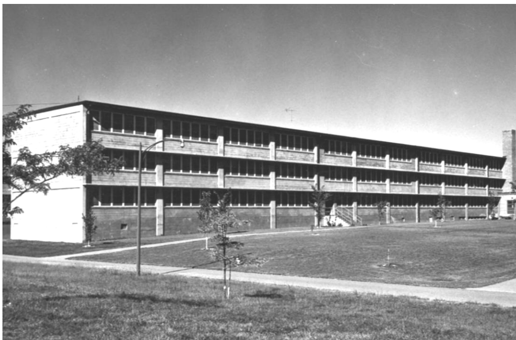
Figure 22. Completed Hammerhead barracks, mid-1950s (Museum Division, Fort Riley).
