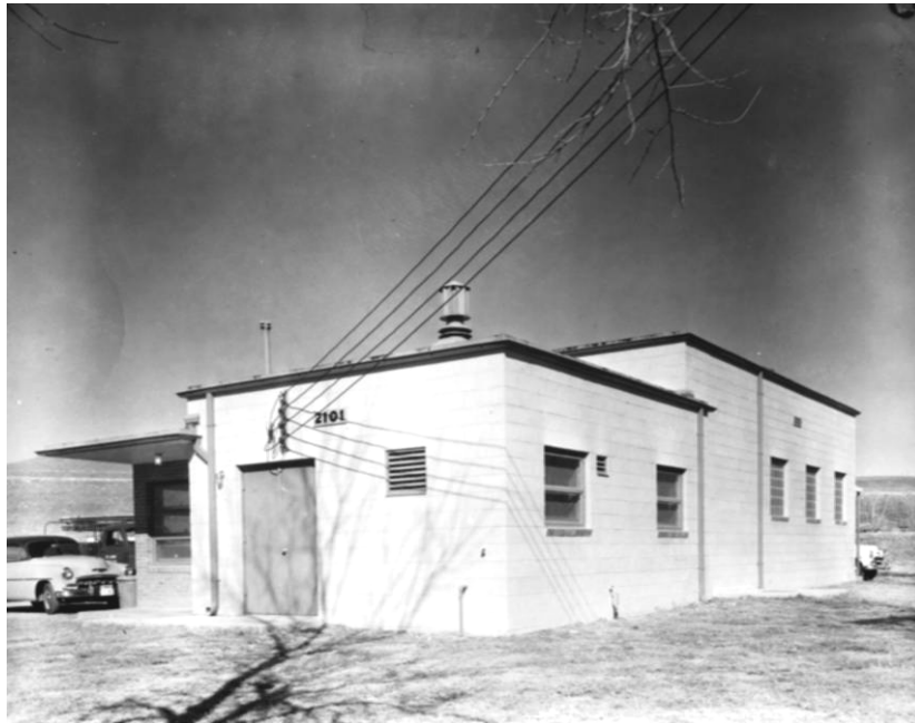
Figure 19. Building 2101, new telephone exchange building, Camp Forsyth, 1954 (NARA).
