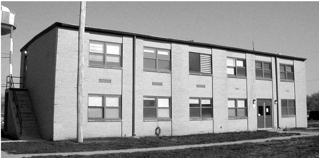
Figure 40. Fort Riley Building 725 (ERDC-CERL 2007).
