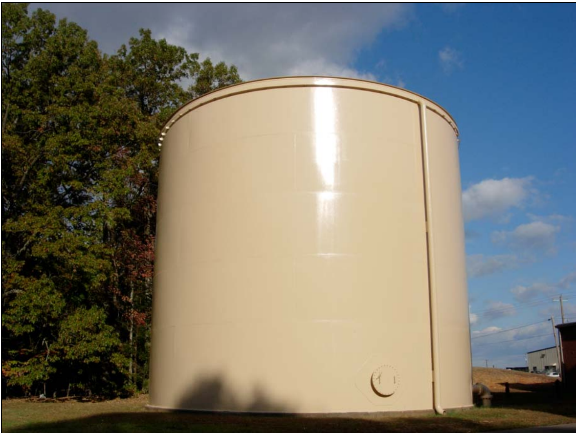
Figure 11: Sabre Deluge Tank after application of the coating system by MANTA
