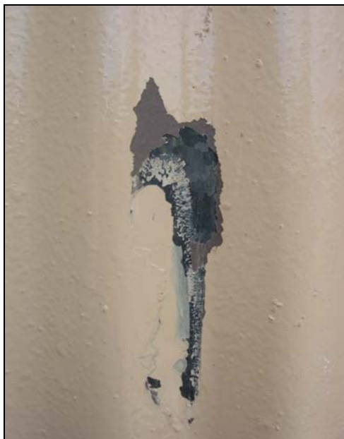
Figure 26: Close-up of area after removal
