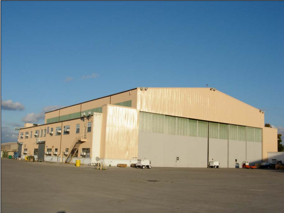
Figure 22: Hangar #2 Ft. Campbell upon Completion
