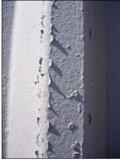
Figure 19: In-Progress Inspection (Hangar#1)
