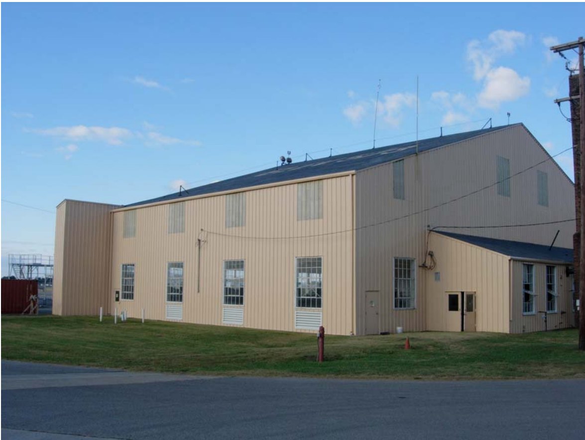
Figure 17: Hangar #1 upon Completion
