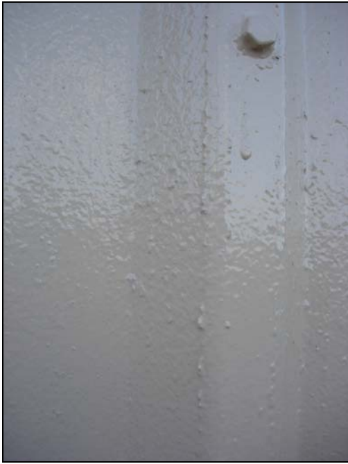
Figure 18: Final Inspection (Hangar #1)
