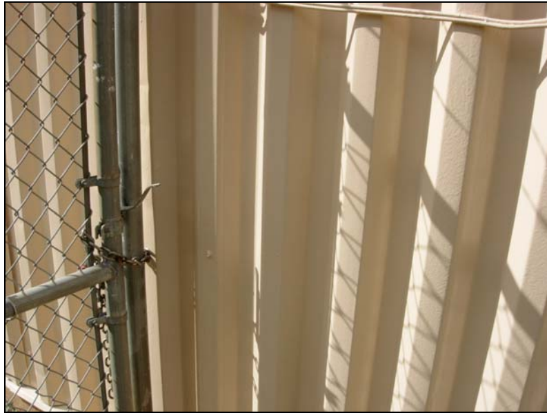
Figure 37: Close-up of the gate and latching device
