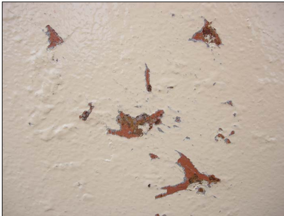
Figure 5: Loose coatings removed with dull putty knife
