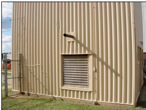
Figure 38: Long view of gate area
