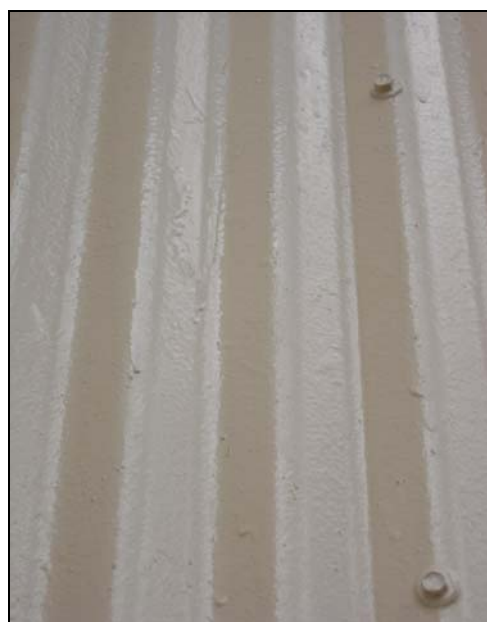
Figure 25: Close-up after repair
