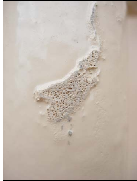
Figure 15: Roller nap removed
