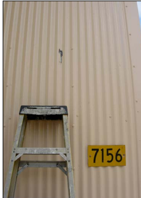
Figure 24: Long view after removal
