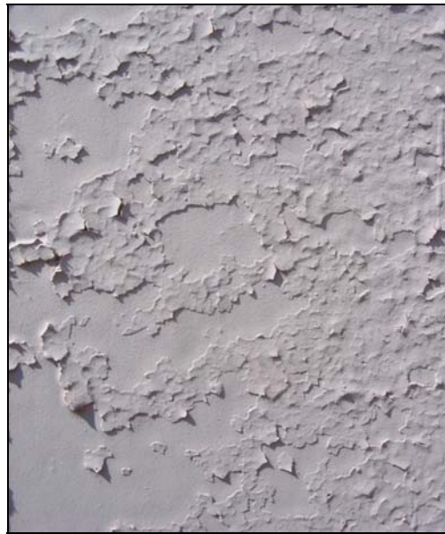
Figure 21: In-Progress Inspection (Hangar#1)
