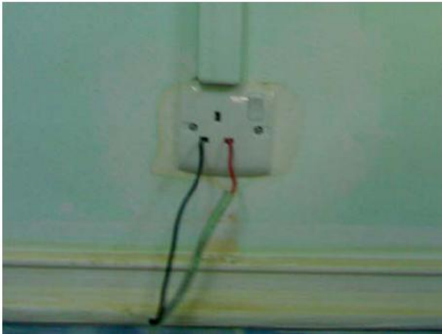
Site Photos 14 and 15. Unsafe electrical practices used by the contractor and captured in daily QA reports (Courtesy of USACE)
