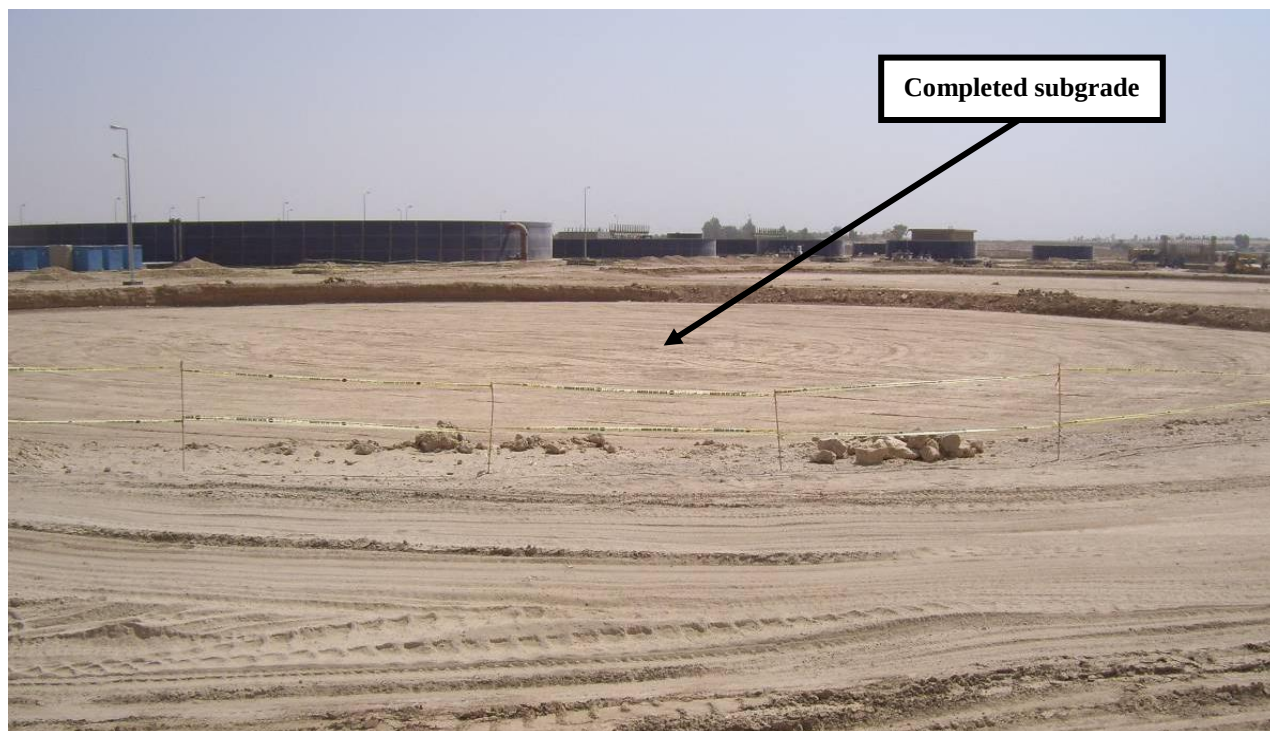
Site Photo 7. Aeration tank subgrade
