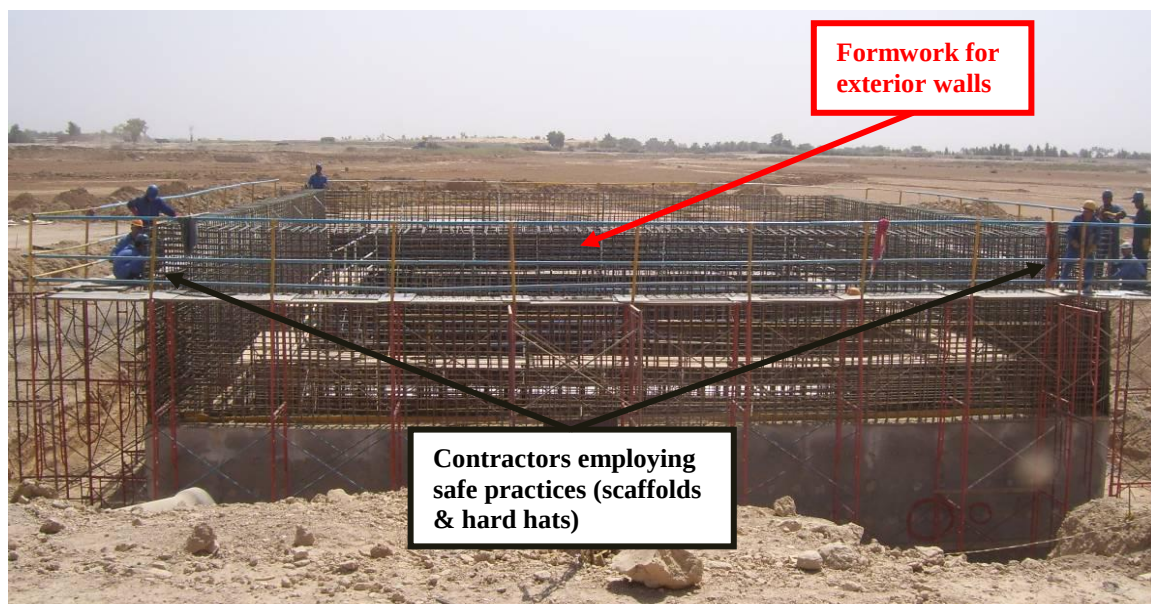
Site Photo 14. Effluent pump station construction
