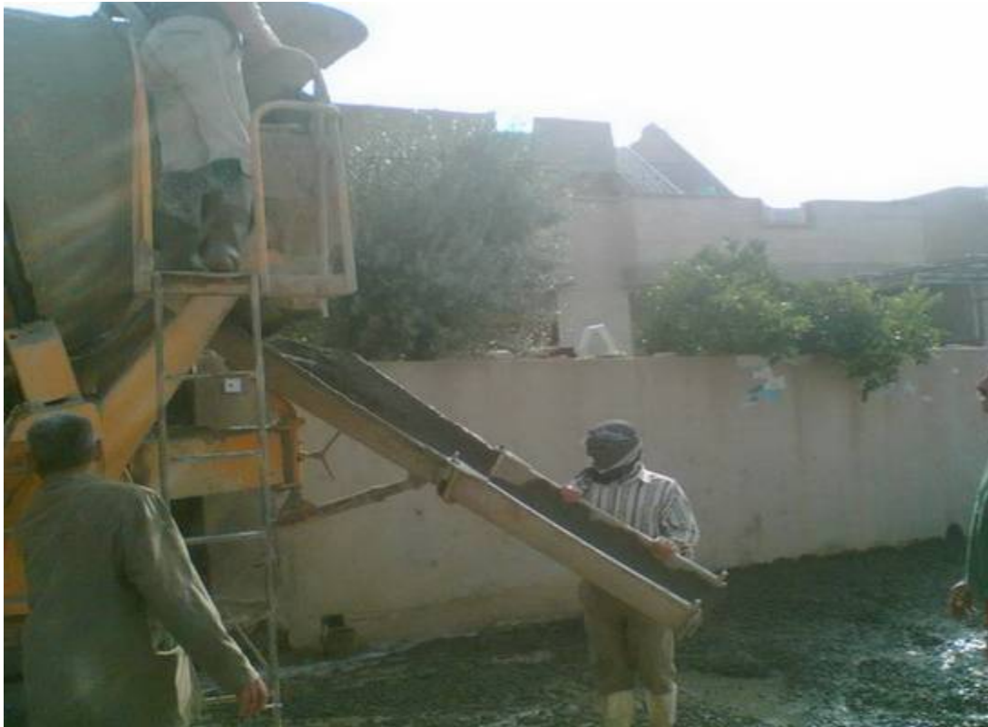
Site Photo 3. Aggregate base and concrete base pour (Photo courtesy of USACE)
