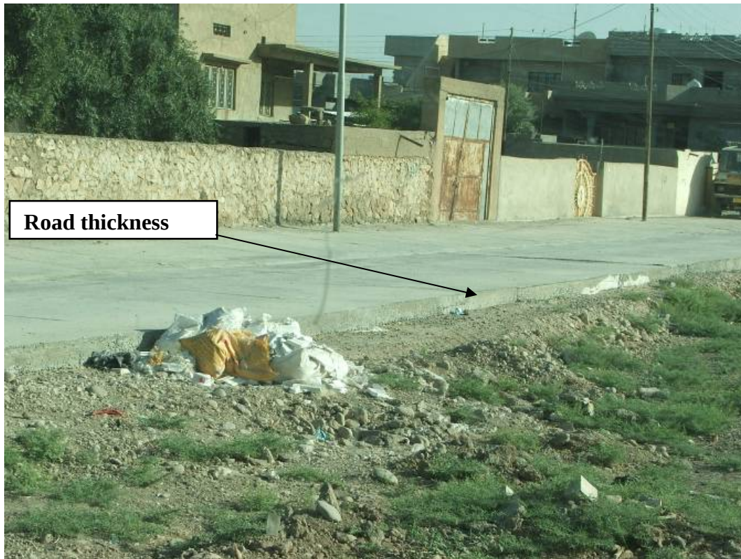
Site Photo 9. Newly constructed road thickness
