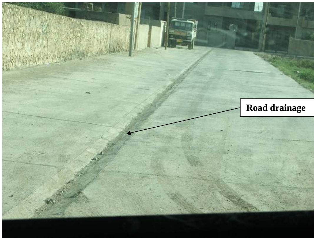
Site Photo 10. Newly constructed road drainage
