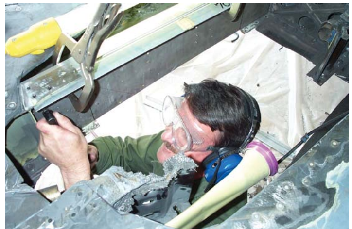
TSgt David Keiser from the AF ABDR Program Office drills holes for the wings internal structural repair.
