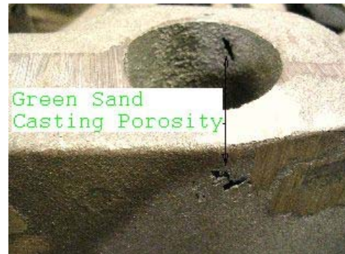
Figure 2-17: Close up of Through Wall Casting Defects
