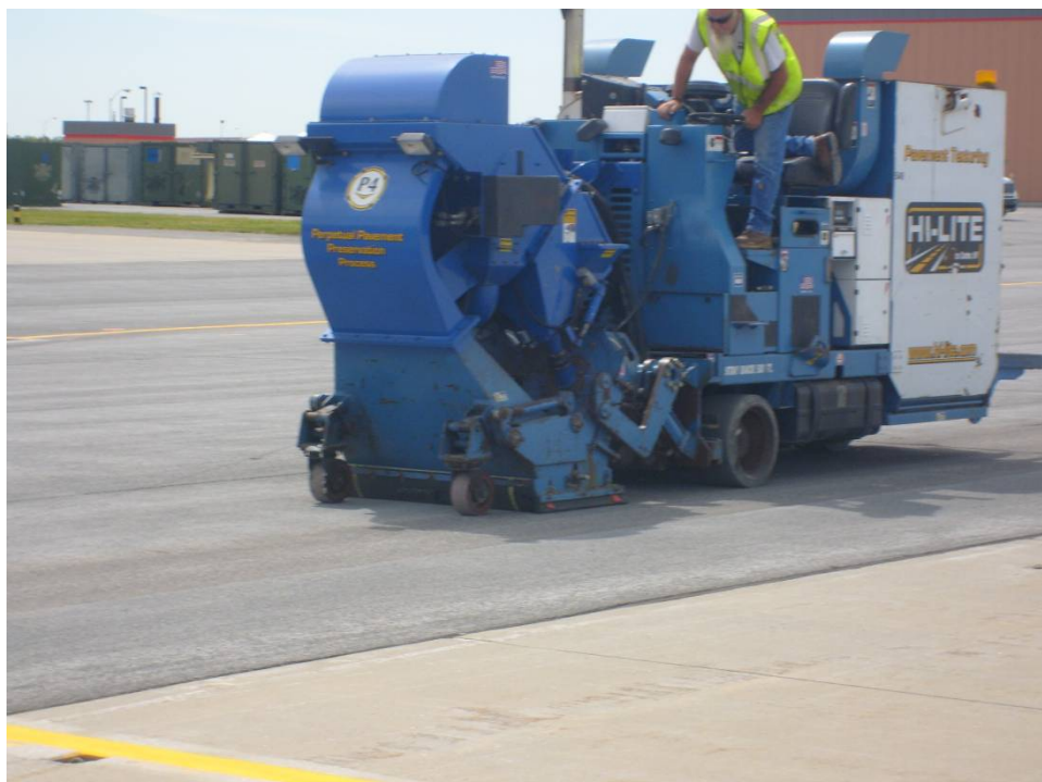
Figure 15. Shot blaster during operation.
