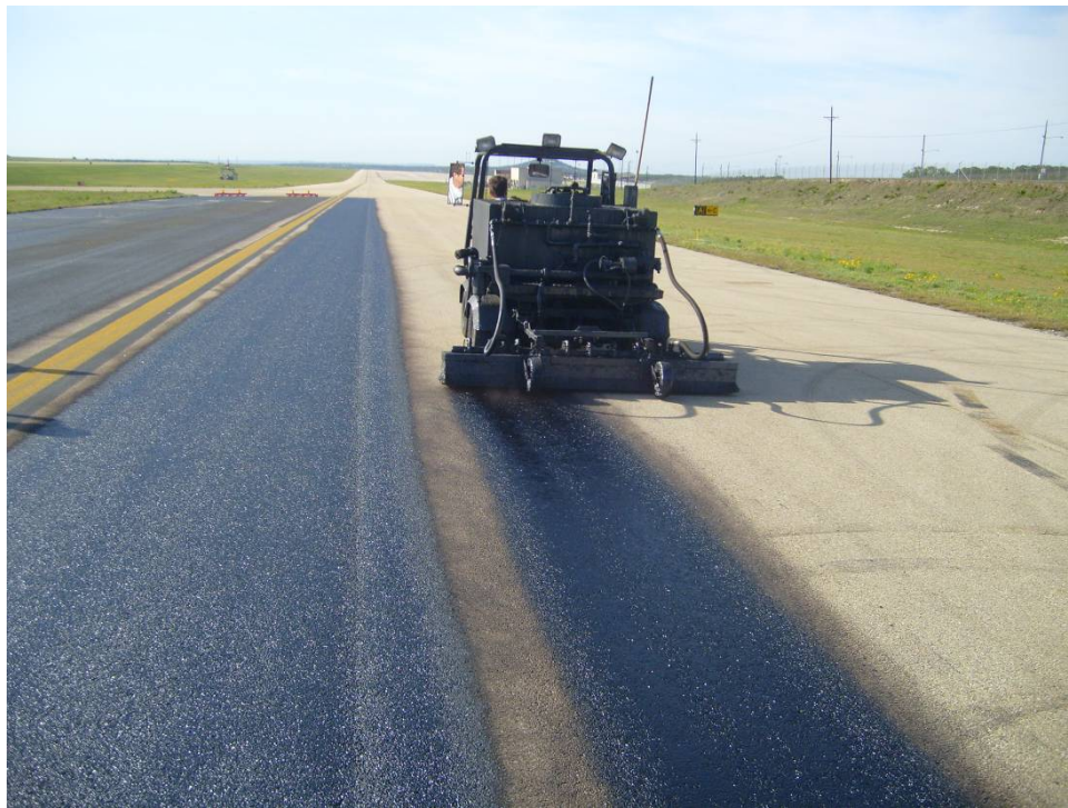
Figure 25. Application of PaverX asphalt rejuvenator.
