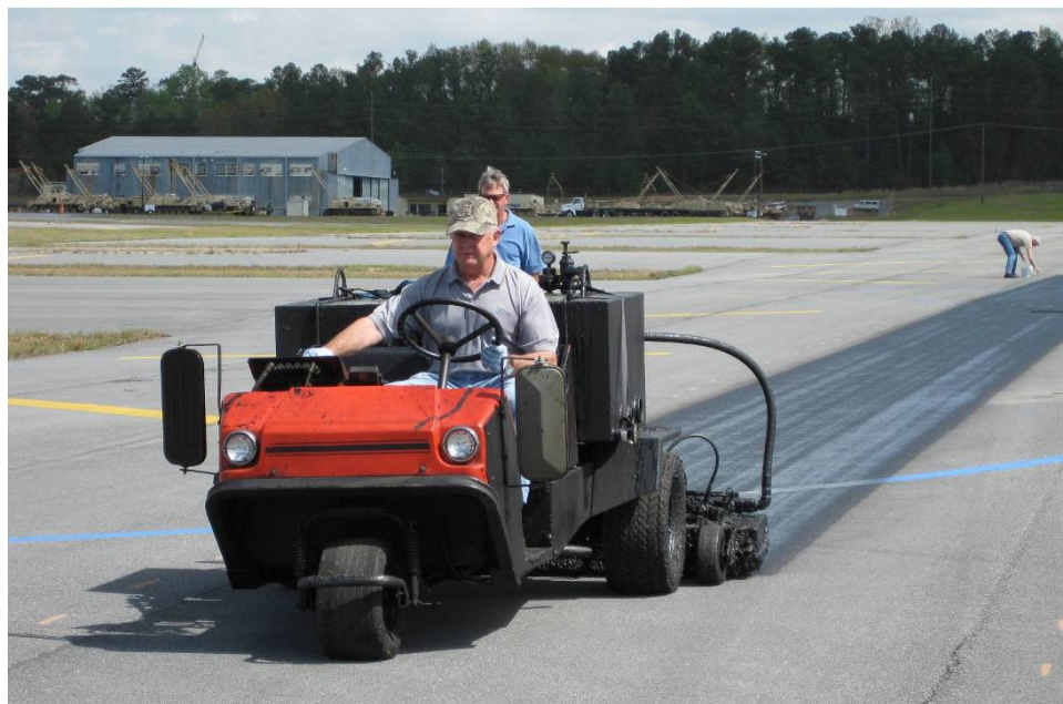
Figure 17. Application of Pavement Dressing Conditioner (PDC).
