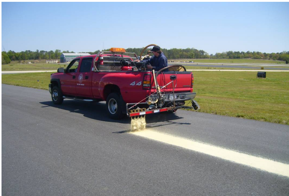
Figure 19. Joint Bond application.
