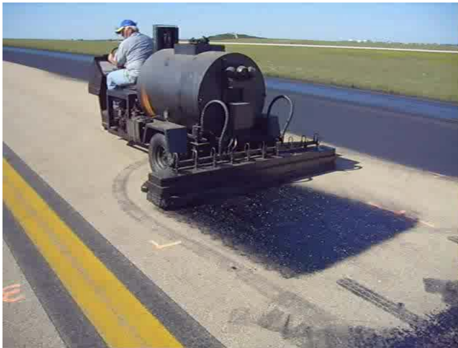
Figure 12. Application of Gem Seal CBRTSO asphalt rejuvenator.
