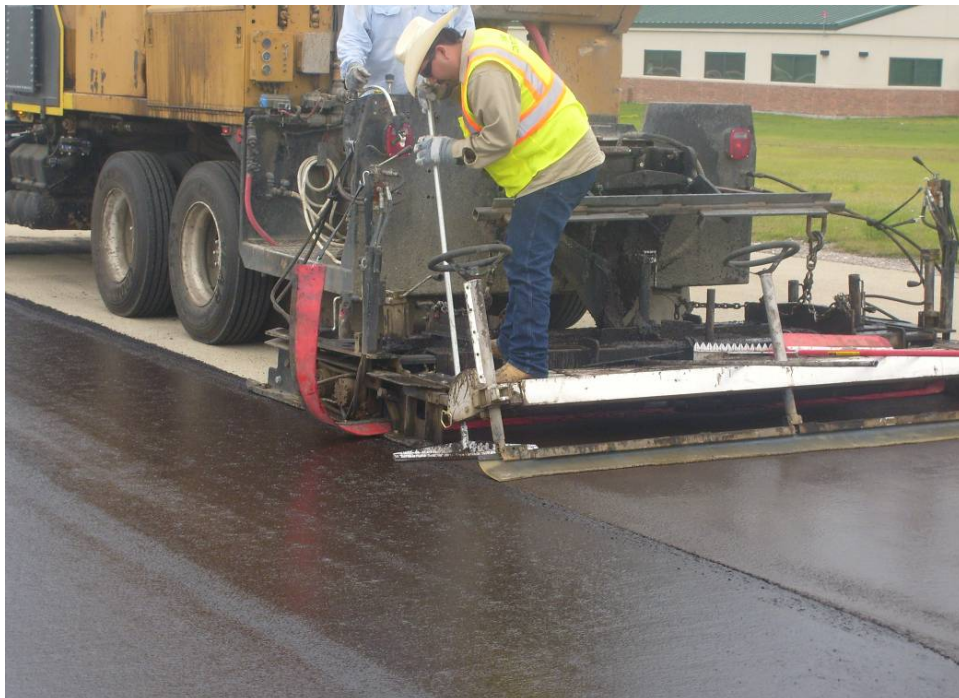
Figure 22. Application of Viking Construction Type II slurry seal.
