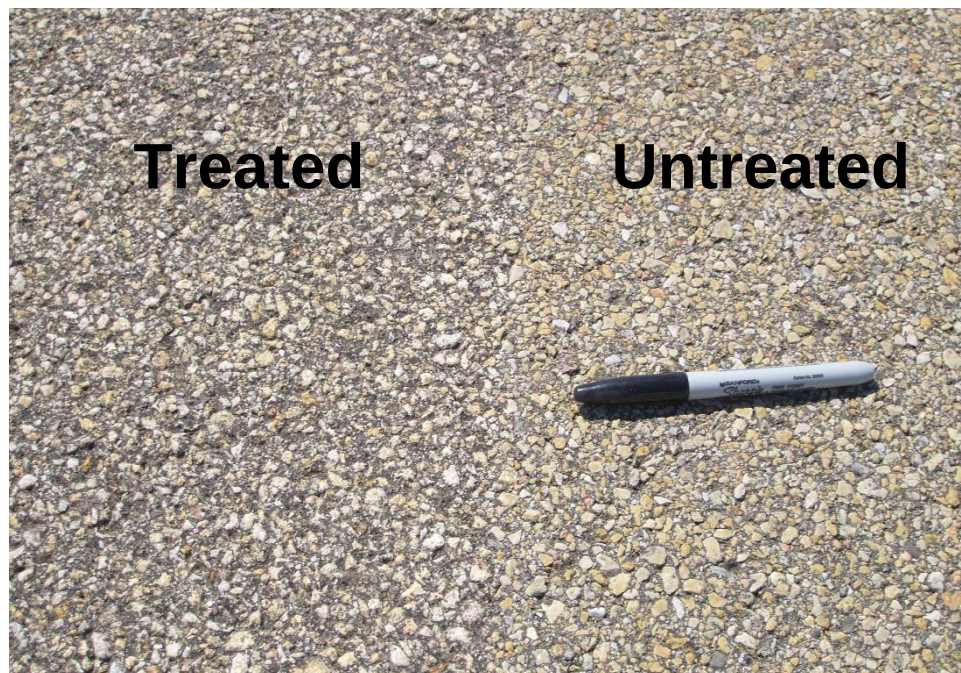
Figure 16. Shot blasted asphalt pavement.
