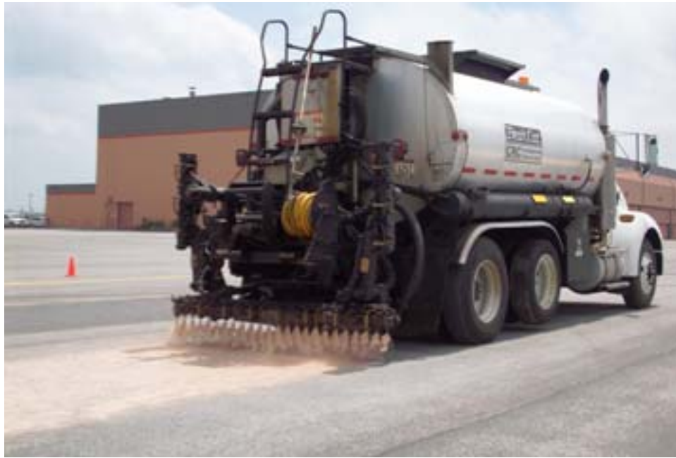
Figure 18. Application of Reclamite.
