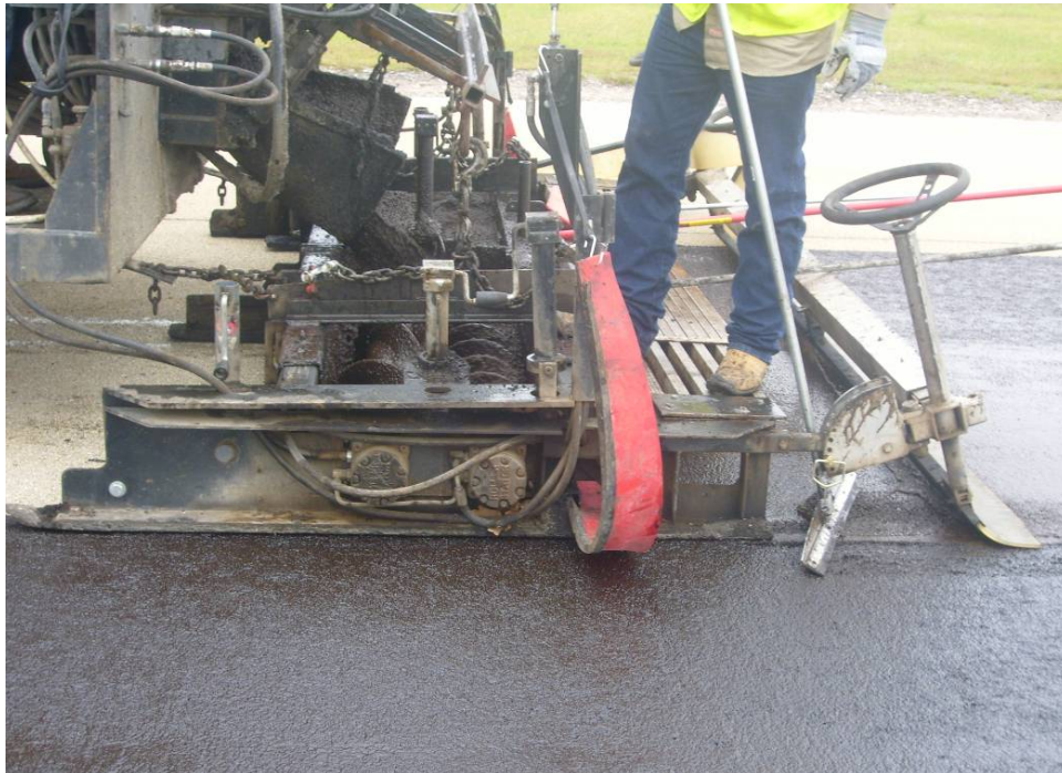
Figure 21. Side view of Viking Construction slurry box.
