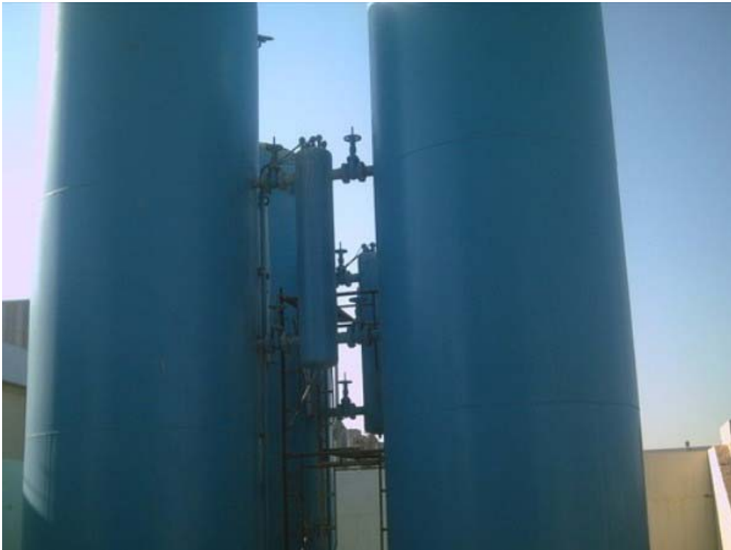
Site Photo 11. Anti-hammer system (Photo courtesy of USACE)
