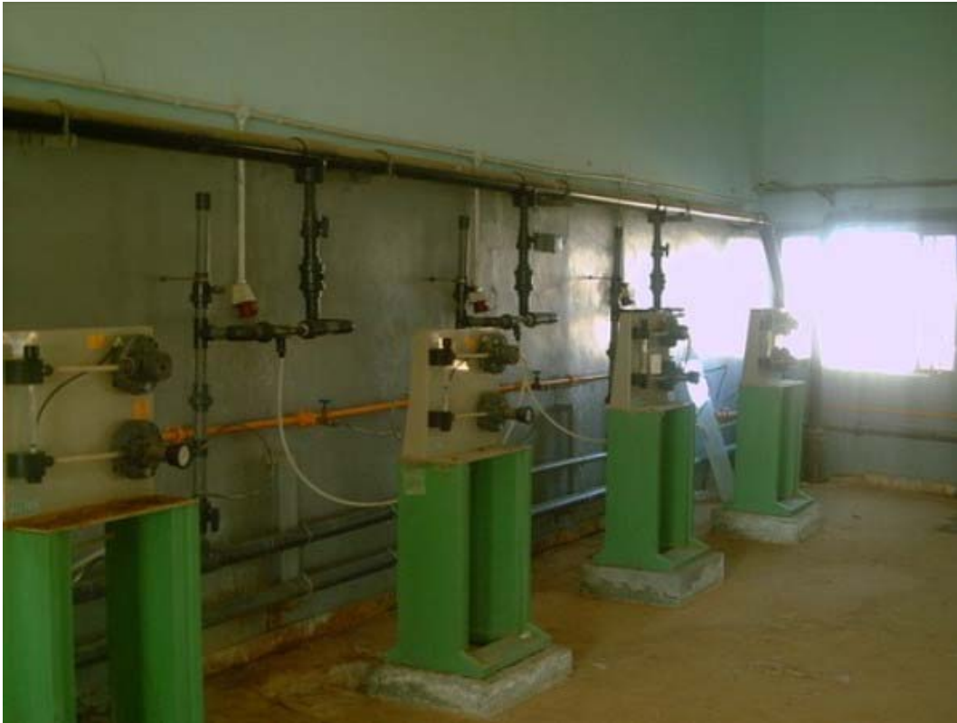
Site Photo 12. Chlorine dosing sets (Photo courtesy of USACE)
