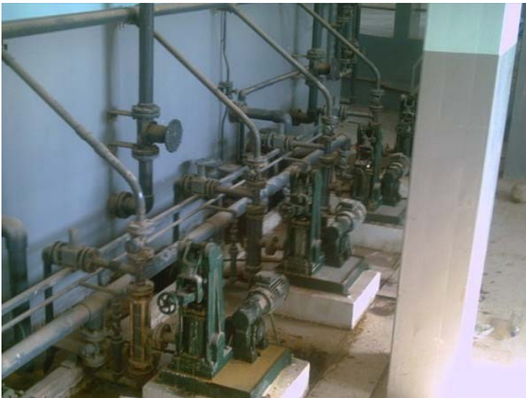
Site Photo 13. Alum mixers (Photo courtesy of USACE)
