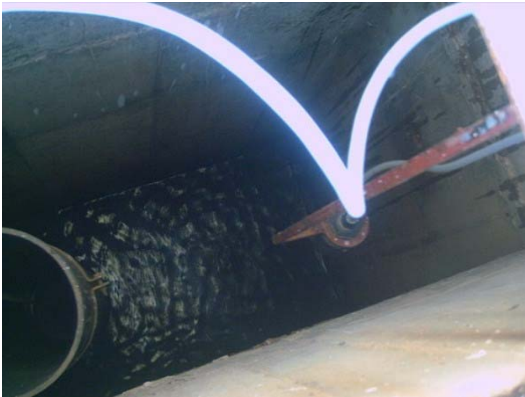
Site Photo 15. Water level indicator (Photo courtesy of USACE)
