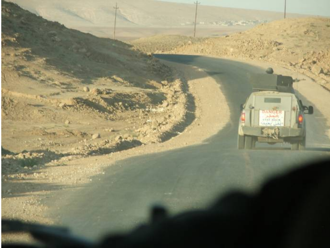
Site Photo 16. New road in use.
