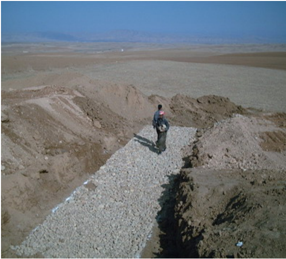
Site Photo 11. Trench excavated for pipe culvert (Photo courtesy of USACE).
