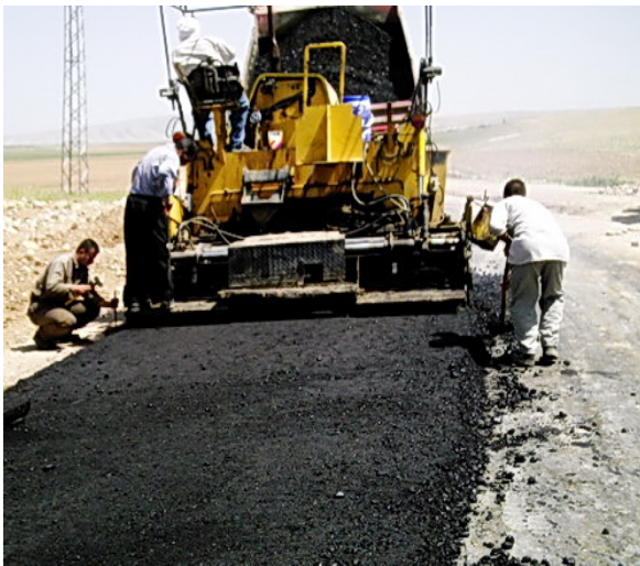
Site Photo 13. Top coat asphalt laying (Photo courtesy of USACE).
