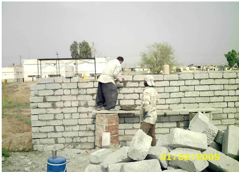
Site Photo 12. Construction of security wall (Photo courtesy of USACE)
