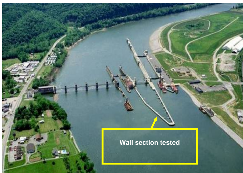
Figure A.1. Winfield Lock and Dam.
