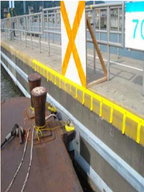
Figure 3.2. Barge with Load Cell Impact at Winfield.
