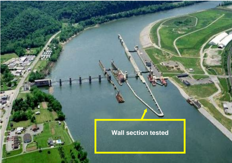
Figure 3.1. Winfield Lock and Dam.
