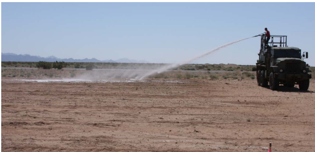
Figure 17. Application of dust palliative using the tower gun method.
