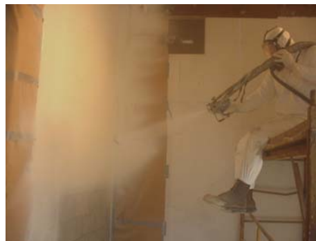
Figure 2. Application of Spray-on Polymer
