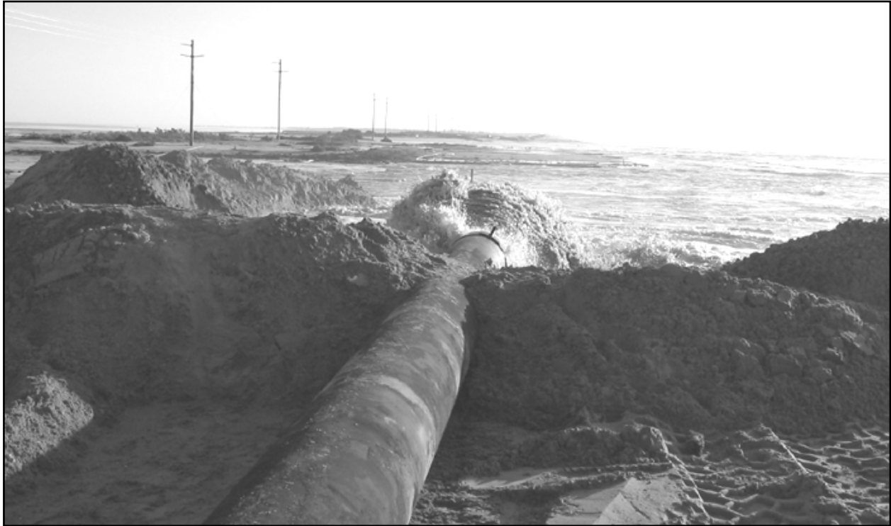
Figure 18. Discharge at western shoulder of breach. View is towards northeast. Island dividing west and center breach channels is in background.
