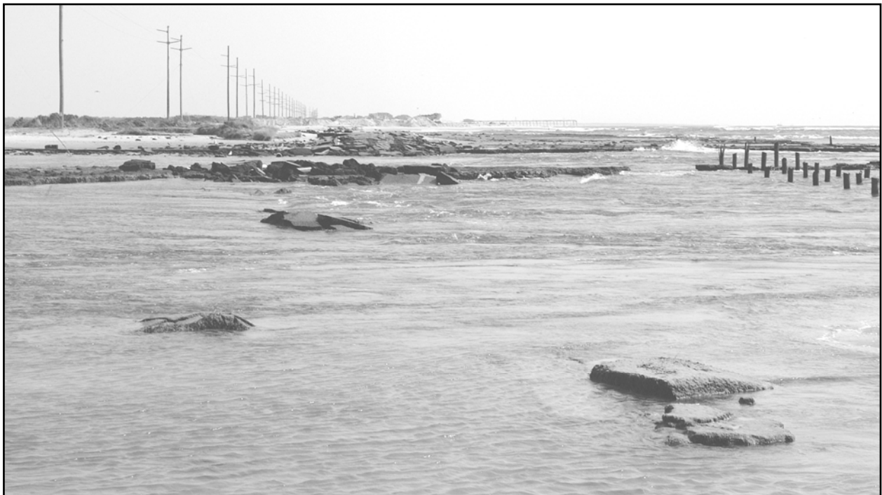
Figure 6. West breach channel, looking east, 5 October 2003. Note old bridge pilings on right and extensive road debris in channel.
