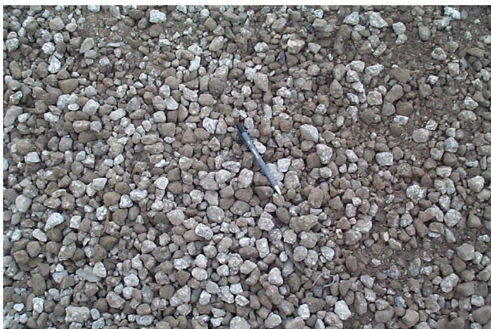
Figure 9. Finished recycled concrete aggregate.
