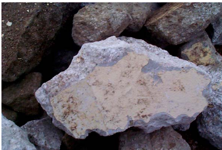
Figure 8. Painted concrete piece.
