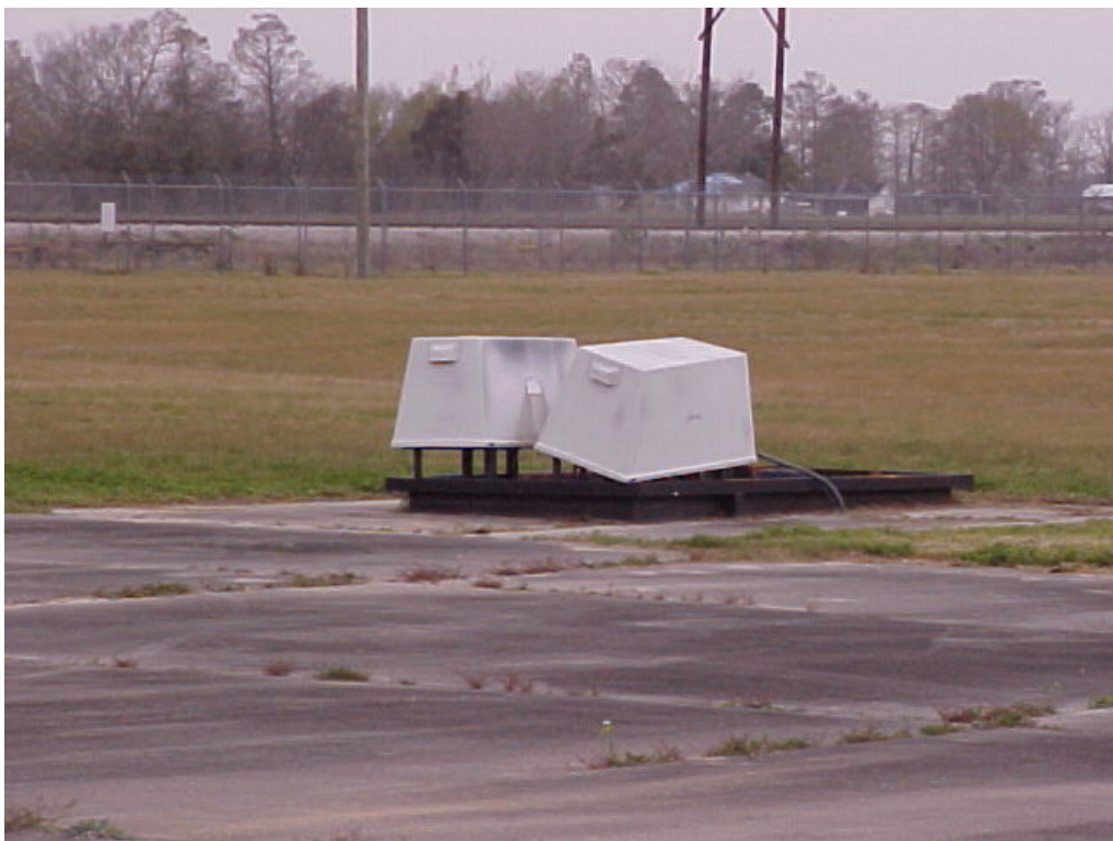
Photograph 68: Wastewater treatment plant. Railroad tracks are visible in background.
