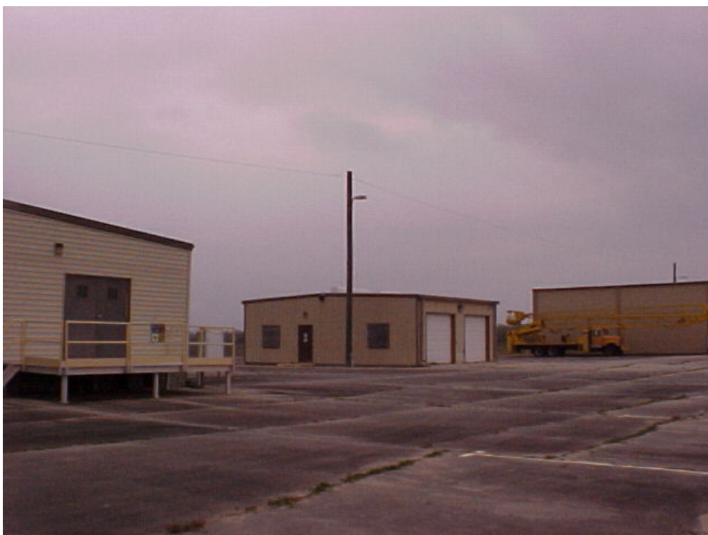
Photograph 4: South wall of Operations Building #001, Mechanical Building #005 and the crane vehicle next to the Payload Service Building #003.
