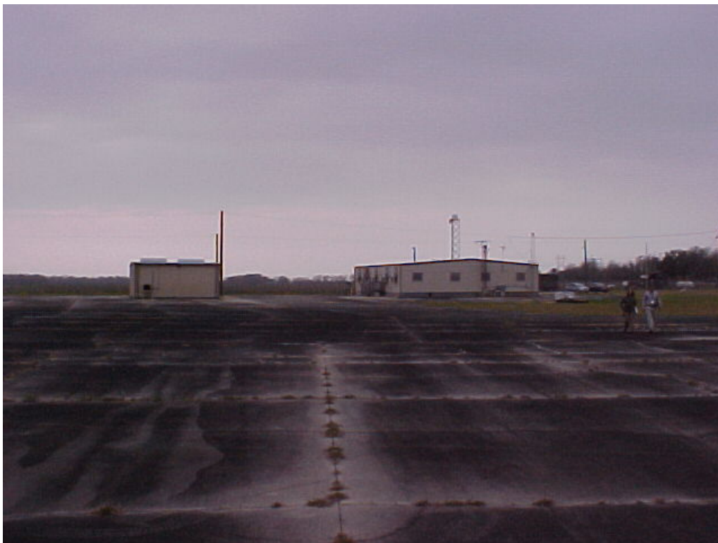
Photograph 31: North side of Mechanical Building #005 and Operations Building #001.
