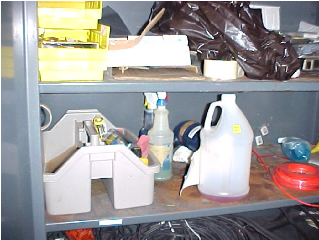
Photograph 40: Miscellaneous maintenance items. Enviro-wash cleaner degreaser, Windex, weed trimmer lines, etc. Mechanical Building #005.
