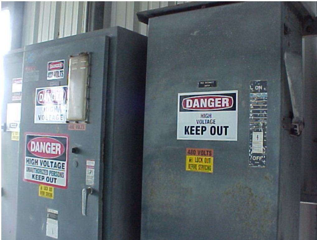
Photograph 65: Transformers located in the Generator Enclosure.
