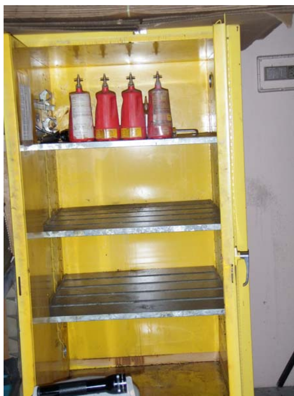
Photograph 44. Flammable storage cabinet in Mechanical Building #005 with nearly empty bottles of methyl ethyl ketone.
