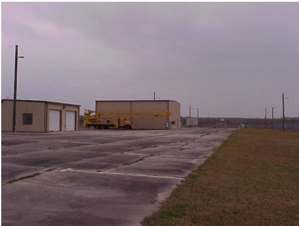
Photograph 29: Mechanical Building #005, Payload Service Building #003, and crane vehicle.
