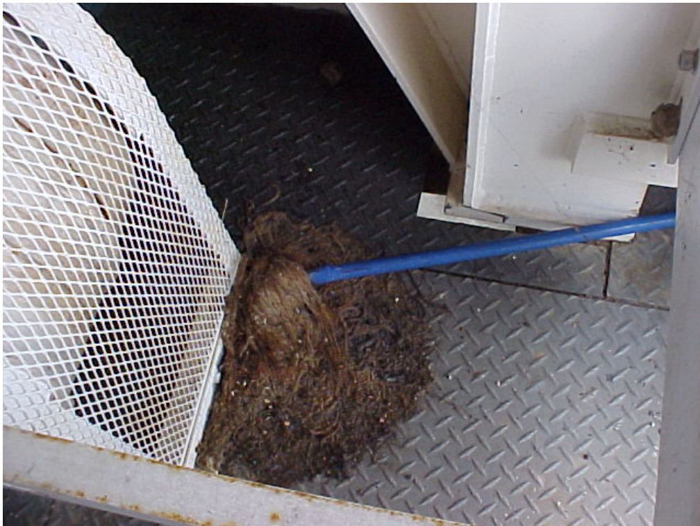
Photograph 78: Old mop located in the Tether Building.
