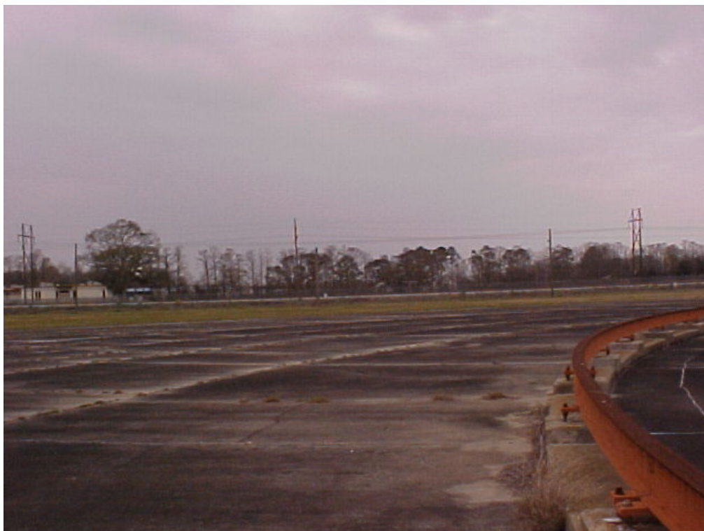
Photograph 76: Launch pad and mooring rail.
