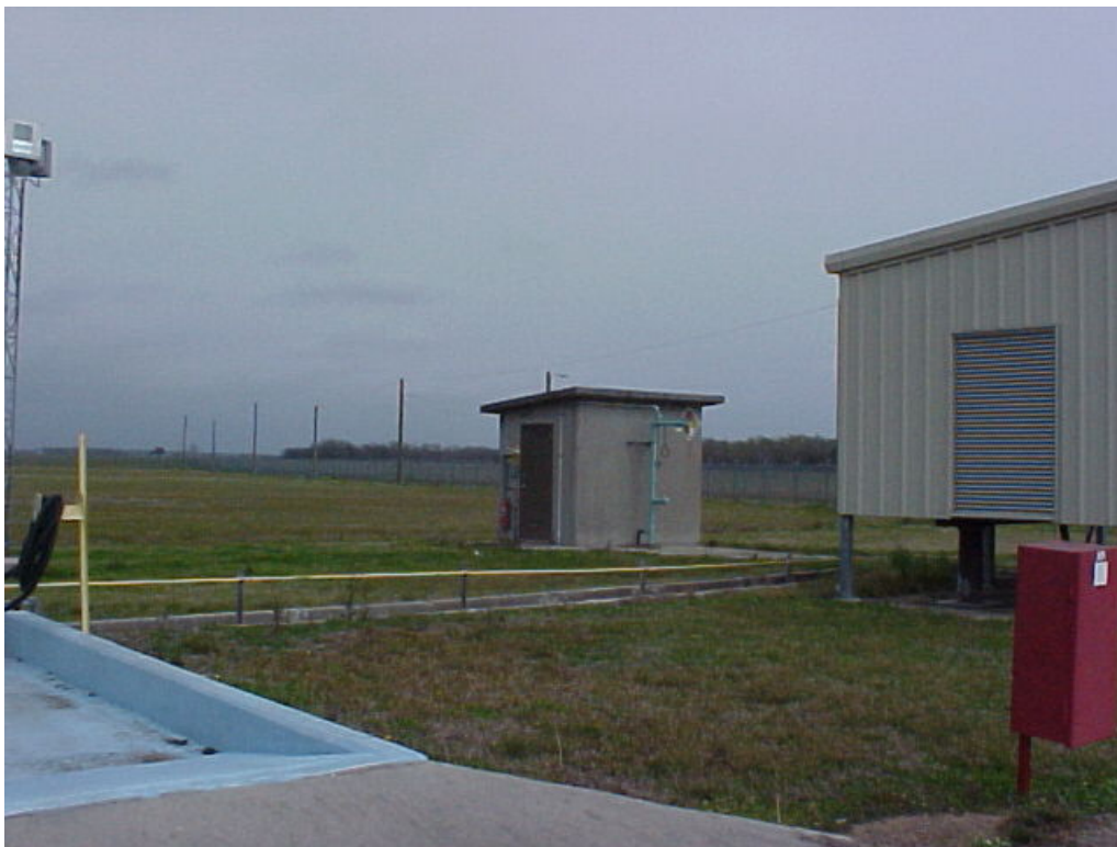
Photograph 67: Front of secondary containment structure (blue), and the yellow aboveground fuel line leading to the elevated Generator Enclosure. The red box contains a fire extinguisher. The Hazardous Material Building #006 is in background.
