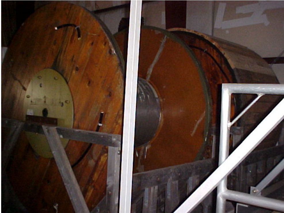
Photograph 49: Large cable reels for the tether. Payload Service Building #003.
