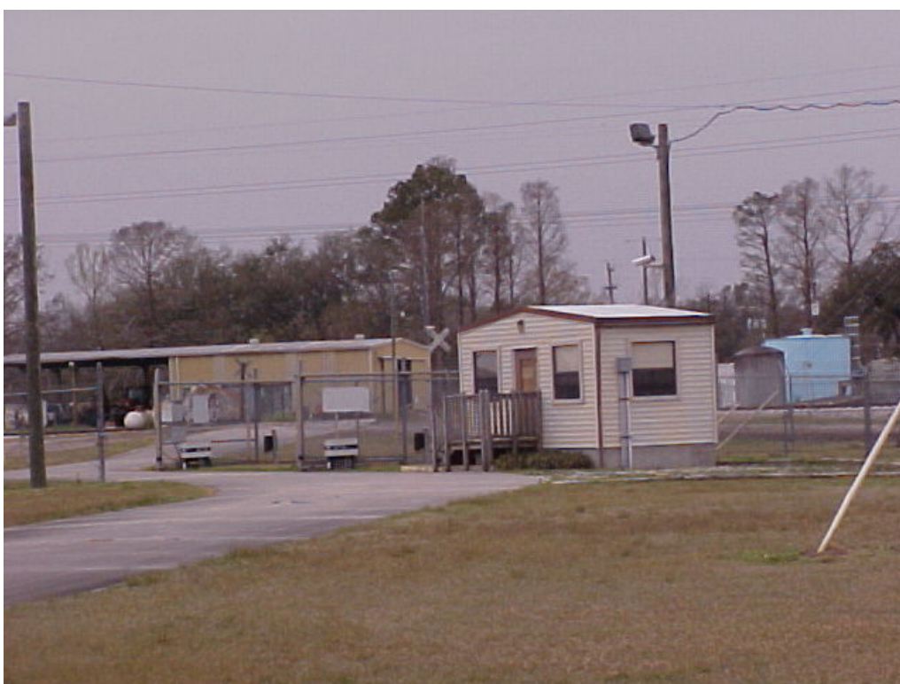
Photograph 2: Closer view of the Guard House and Entry to the TARS Site
