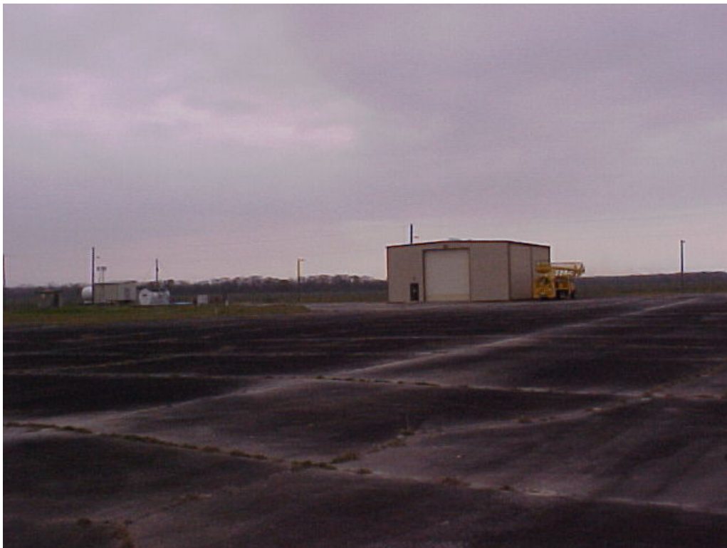
Photograph 46: North side of the Payload Service Building #003.
