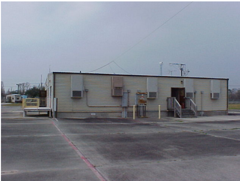
Photograph 7: East wall of the Operations Building #001 showing air conditioning units and transformer box. Guard house is in background.
