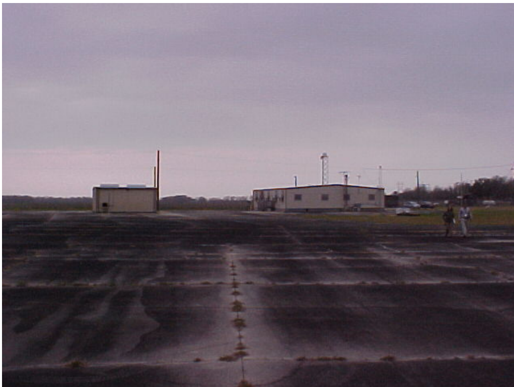
Photograph 6: North side of Mechanical Building #005 and Operations Building #001.
