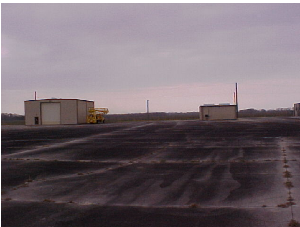
Photograph 30: North side of Payload Service Building #003 and Mechanical Building #005 looking southward.
