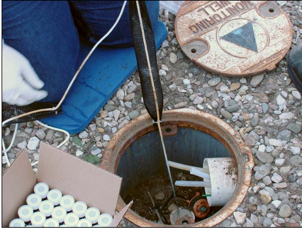
Figure 5-6. Removal of diffusion sampler from a well prior to sampling
