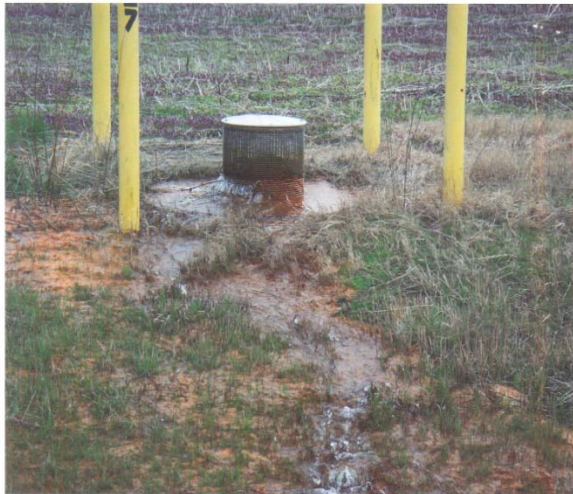
Figure 2. St. Francis River Basin Relief Well
