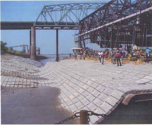
Figure 1. Mississippi River Revetments Project
