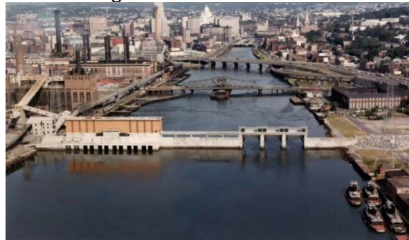
Figure 2. Fox Point Barrier
