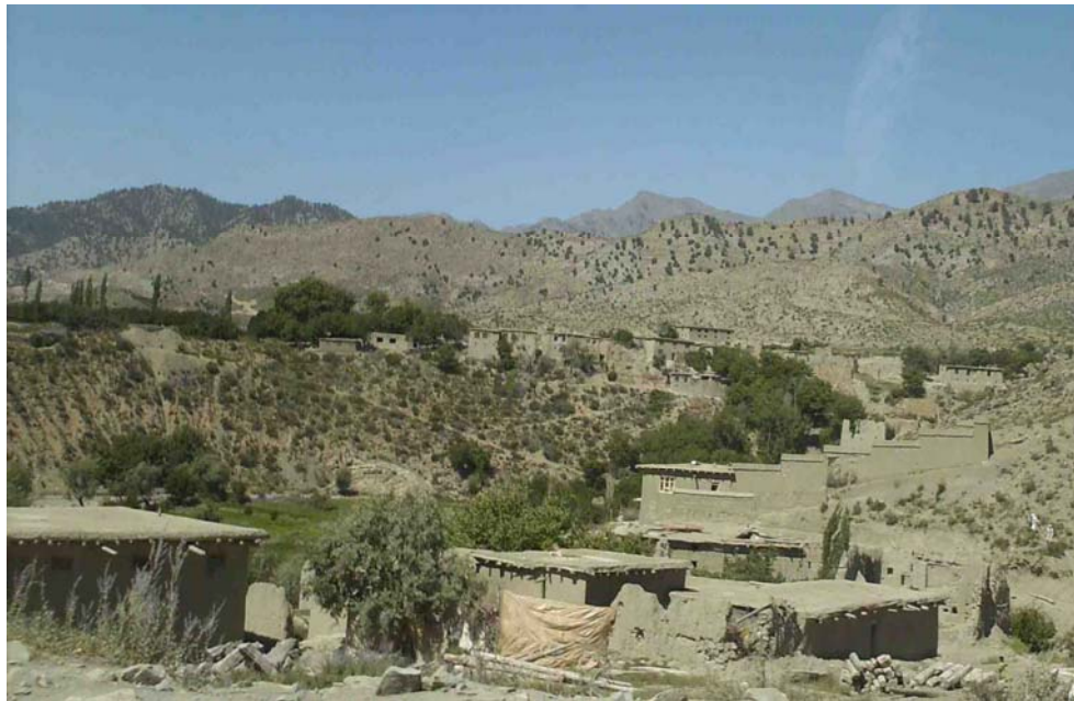
Photo 3. Flat Roof Construction in Khost 297
