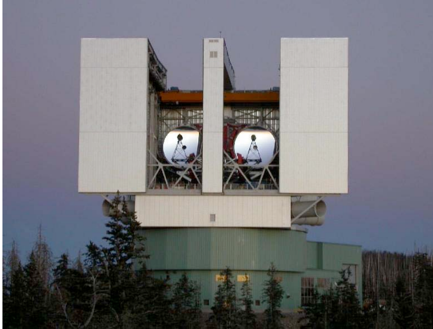
Fig. 1. The Large Binocular Telescope on Mt. Graham, AZ comprises two unit telescopes on a single mount. Each primary mirror is 8.4 m in diameter, and the two unit telescopes can be combined to produce images exactly as would be seen from a single 23 m aperture masked with two 8.4 m holes.
