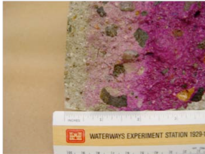
Figure 11. Core sample after application of phenolphthalein.
