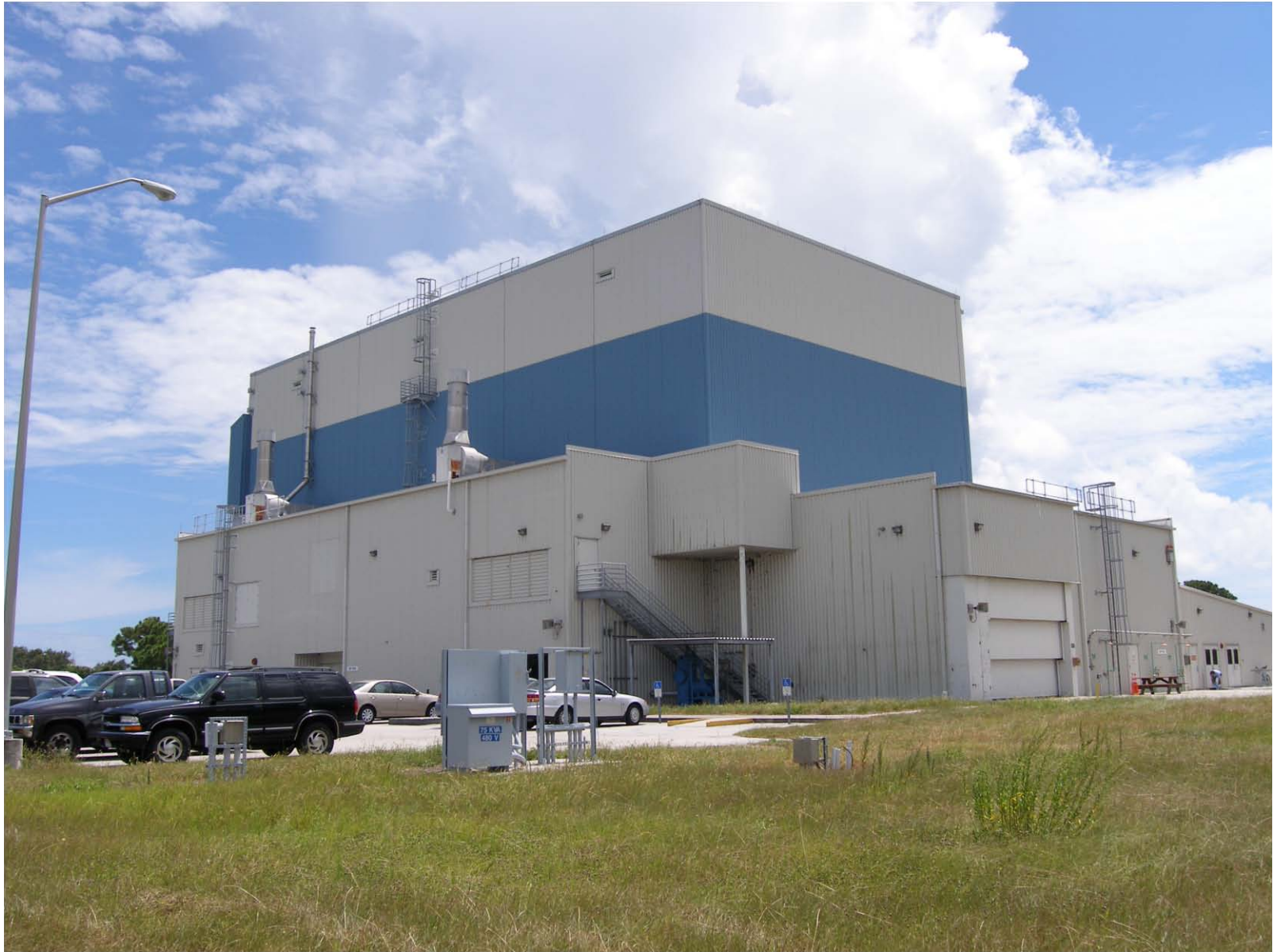
Figure 1. Multi-Payload Processing Facility (MPPF)
