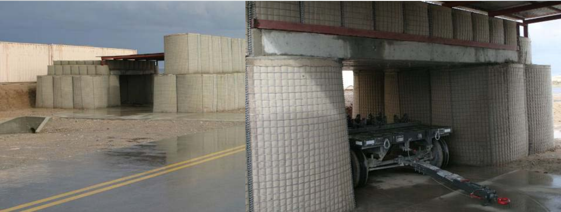
RSB (Ready Storage Building)
