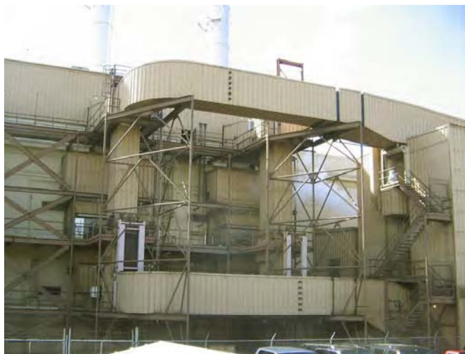
Figure 1. Building 227 exterior before coating application.
