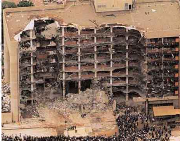
Murrah Federal Building
