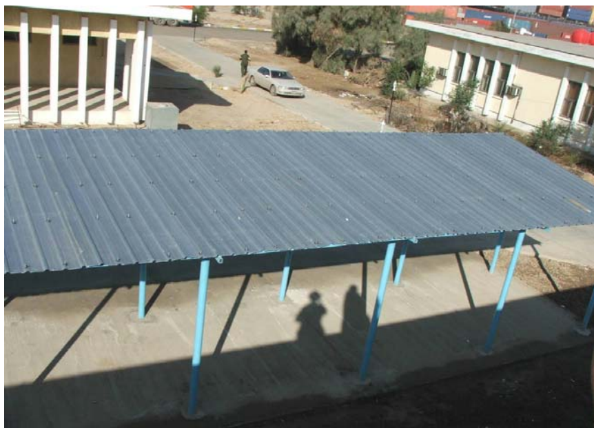
Site Photo 13. Concrete Driveway with Covered Parking
