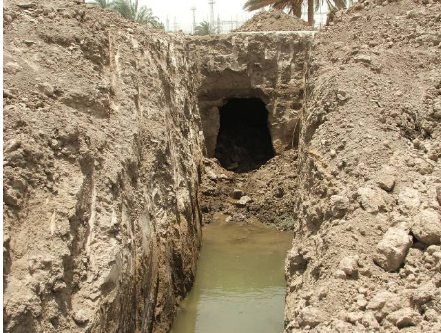
Site photo 4: Point B excavated tunnel under irrigation canal
