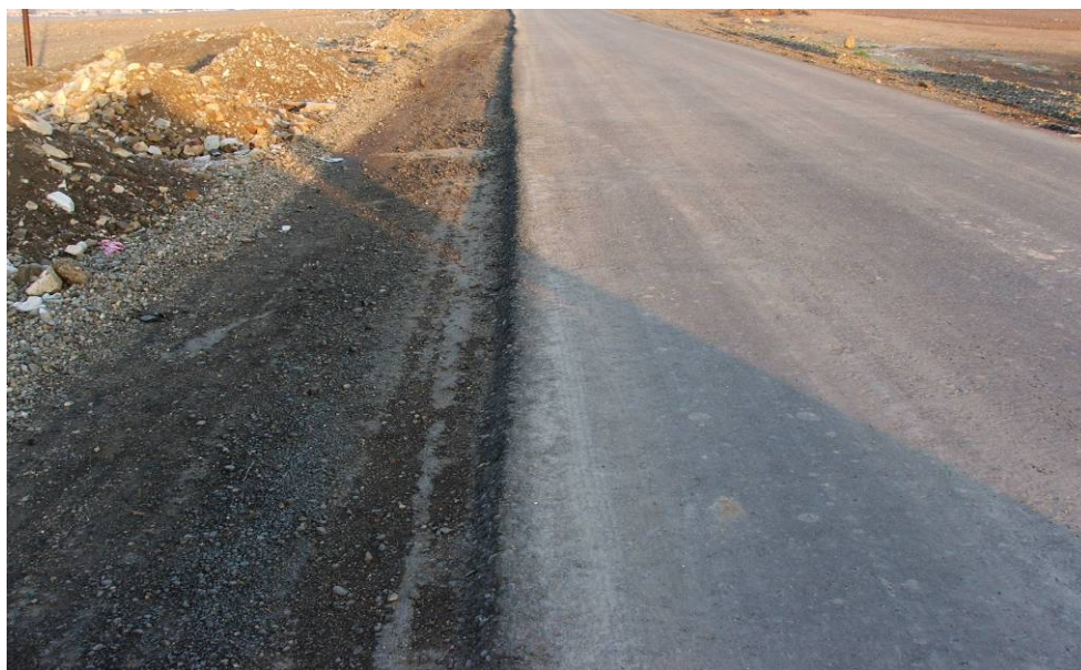
Site Photo 9. Compacted shoulder sub-base
