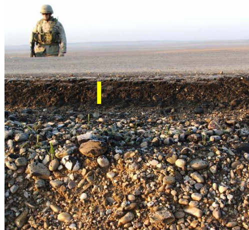
Site Photo 7. Location of measurement
