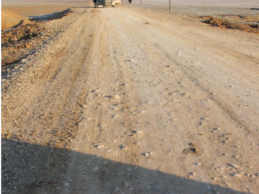
Site Photo 4. Compacted sub-base south of the village of Balawat
