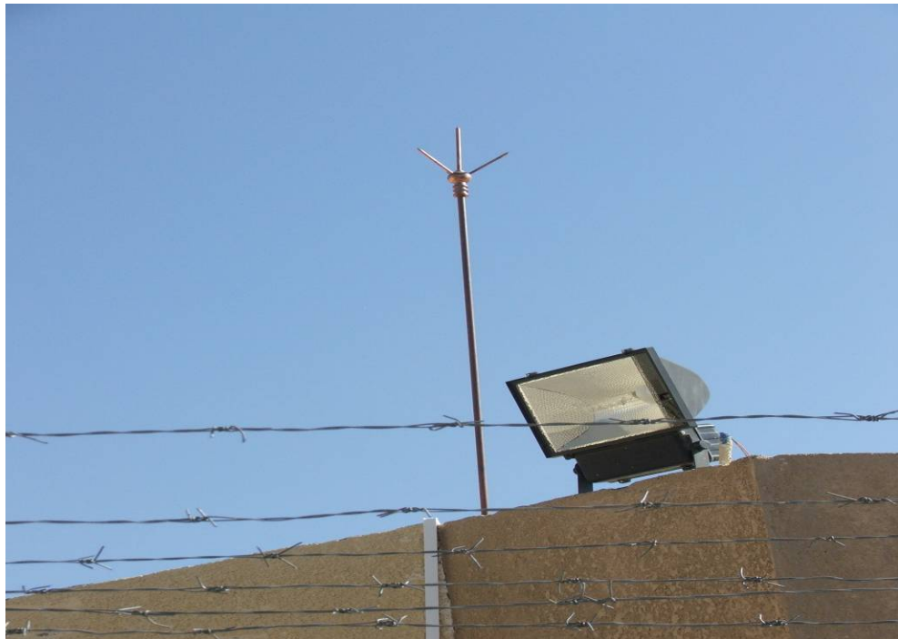
Site Photo 6. Lightning Arrestor and Roof Mounted Light
