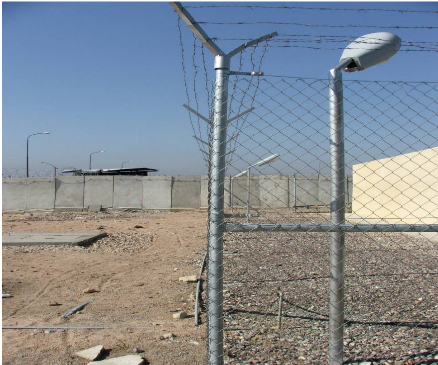
Site Photo 4. Three Pole Mounted Lights on Side of ASP
