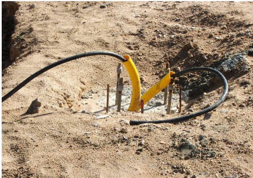
Site Photo 8. Concrete Footers for Perimeter Lighting
