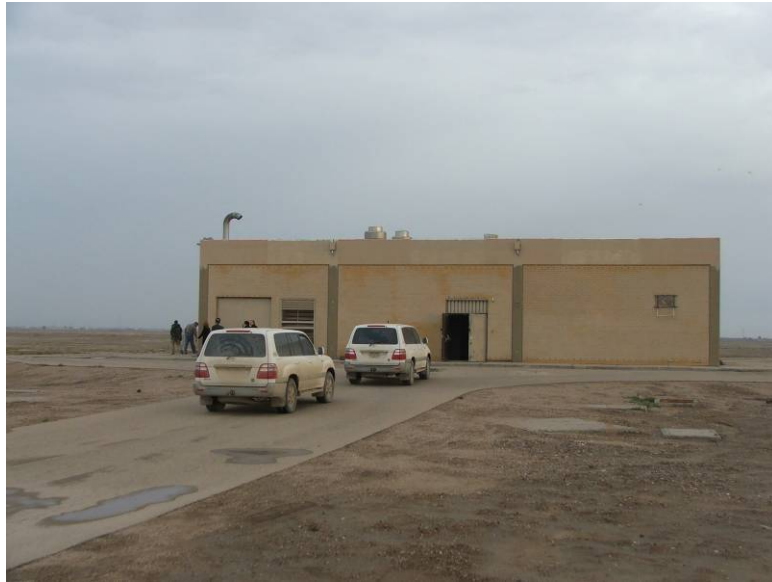
Site Photo 3: Exterior view of S-330 substation
