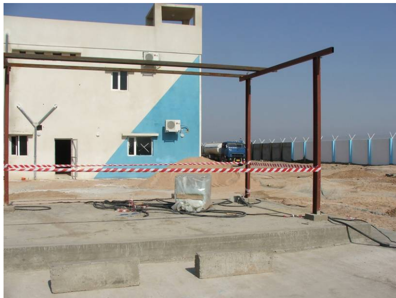
Site Photo 17: Concrete pad for generator unit
