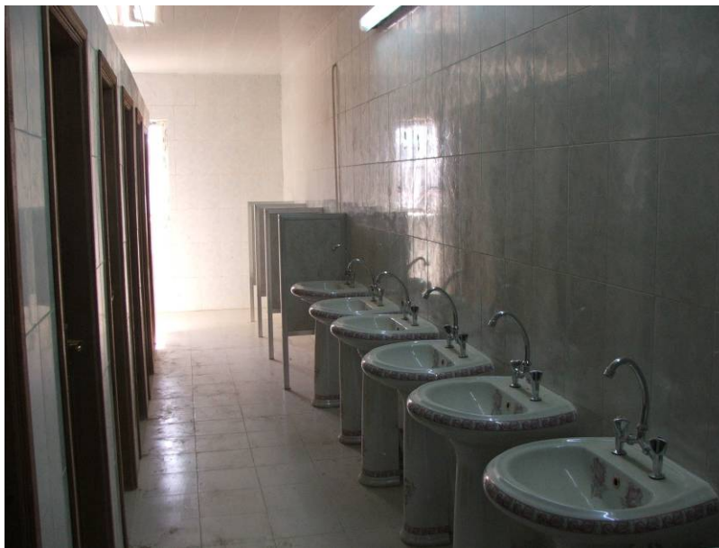
Site Photo 4: Bathroom facility
