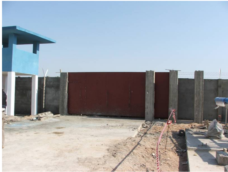
Site Photo 8: Rear entrance gate
