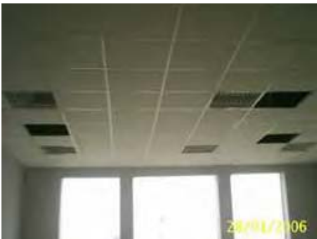
Site Photo 58: Suspended ceilings (Project 11913)
