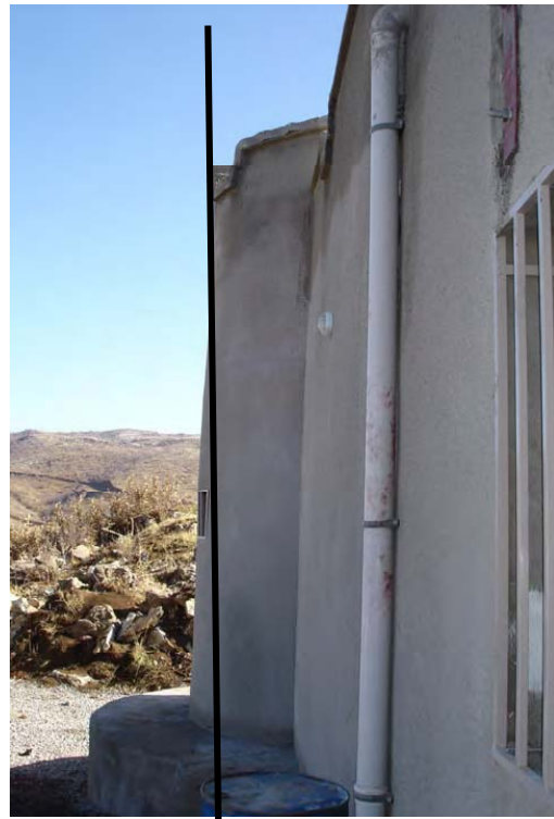
Site Photo 14: Front exterior view showing inward curvature of wall (Project 12831)
