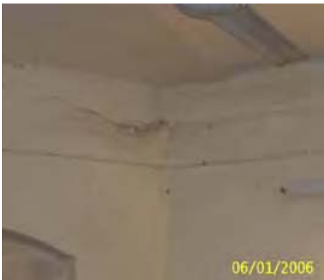
Site Photo 78: Cracks and peeling paint in walls and ceiling (Project 19227)
