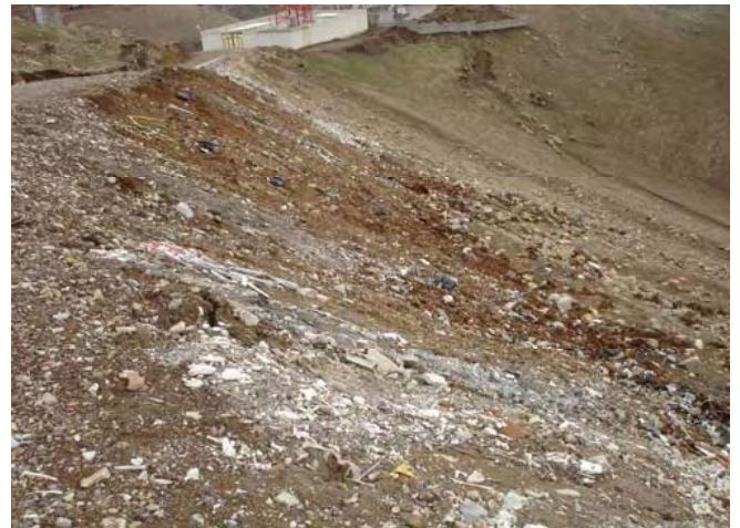
Site Photo 6: Down gradient slope with signs of lateral movement (Project 12807)
