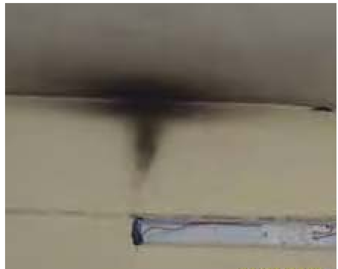
Site Photo 73: Interior electrical light with smoke damage (Project 19179)
