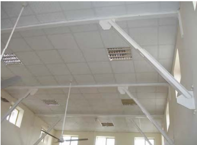
Site Photo 5: Completed structural retrofit (Project 12807)
