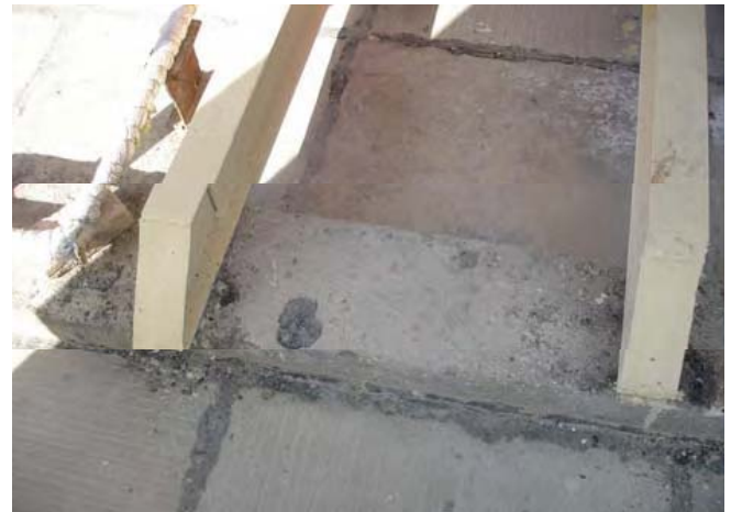
Site Photo 23: Roof mounted water tank base (Project 12855)
