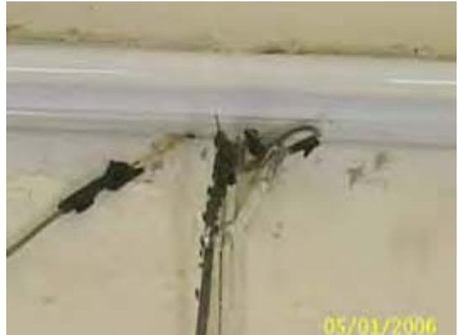
Site Photo 75: Interior electrical light with exposed wiring (Project 19181)
