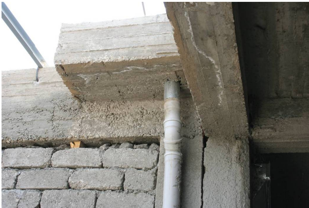
Site Photo 24. Bottom side view of collection basin showing positive rainwater drain piping.
