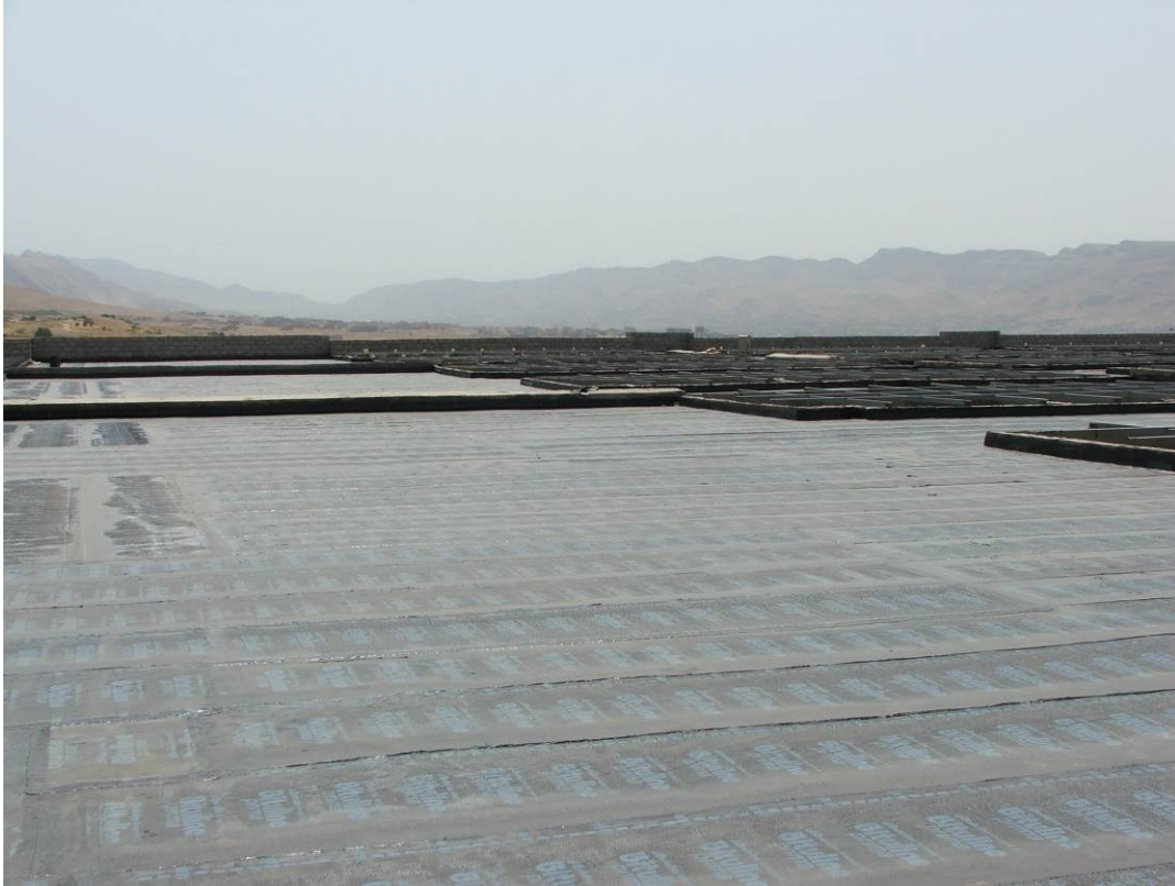
Site Photo 4. Large scale view of bituminous waterproofing membrane.
