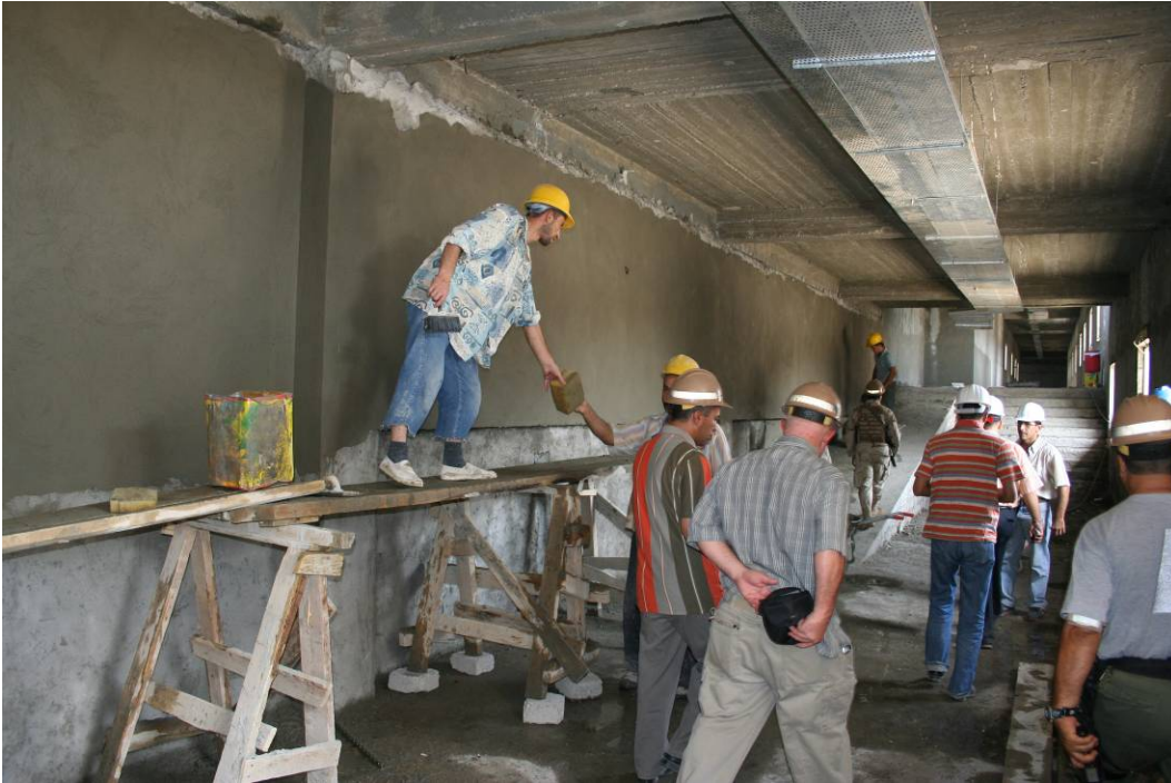
Site Photo 10. Workers finish an interior wall with a thin layer of concrete (plaster).
