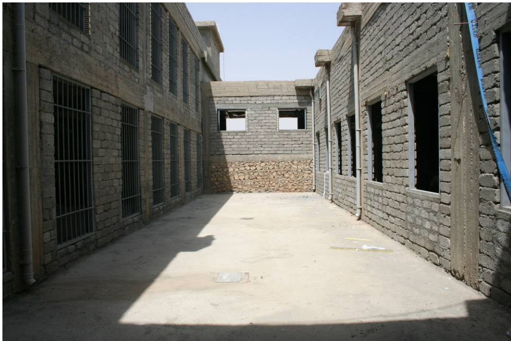
Site Photo 6. Ground floor installation of security protection bar assemblies.
