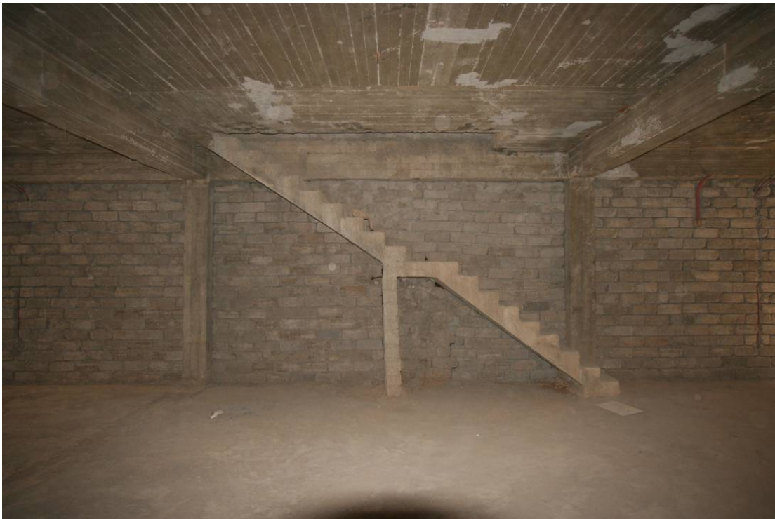
Site Photo 9. Pre-finish side view of poured concrete stairs.
