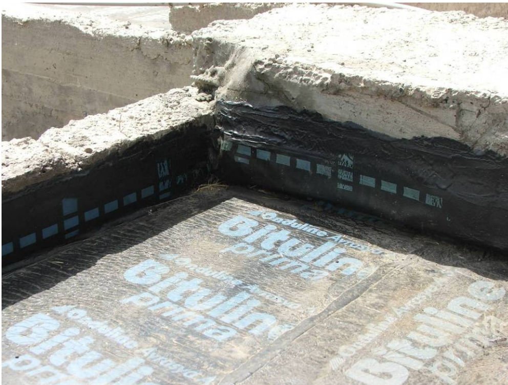
Site Photo 3. Bituminous waterproofing membrane.
