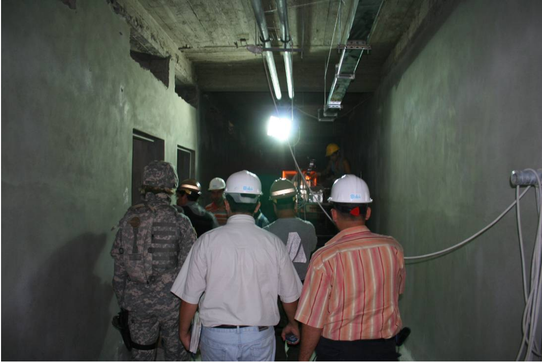
Site Photo 11. Concrete finished interior walls.
