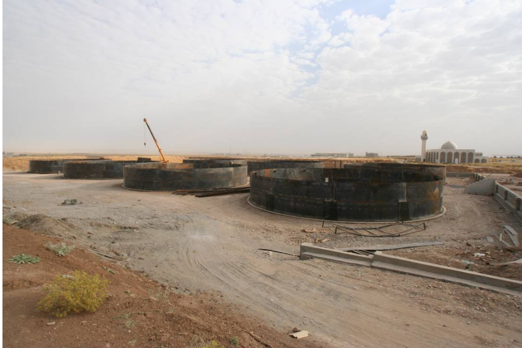
Site Photo 25. Overall construction progress as of 1 August 2006.
