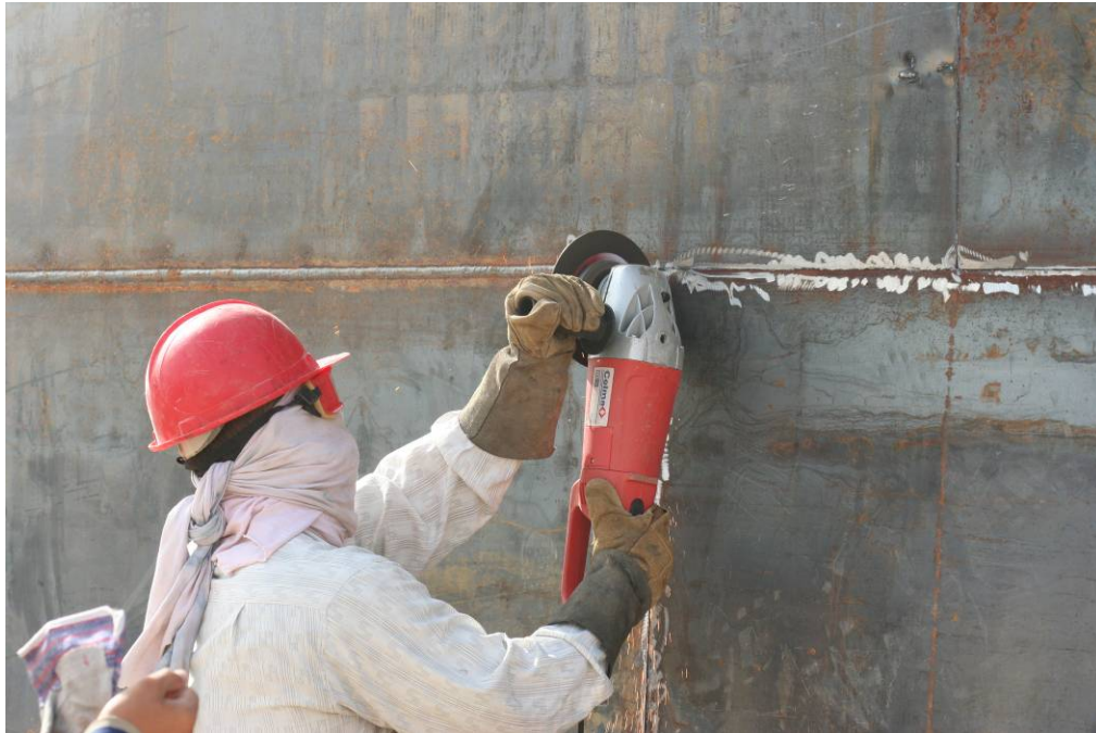
Site Photo 20. Grinding the outside weld back to the shell plating.
