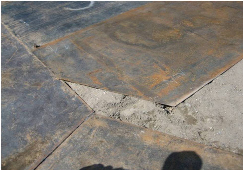
Site Photo 6. Sheets of steel were fitted together prior to welding.
