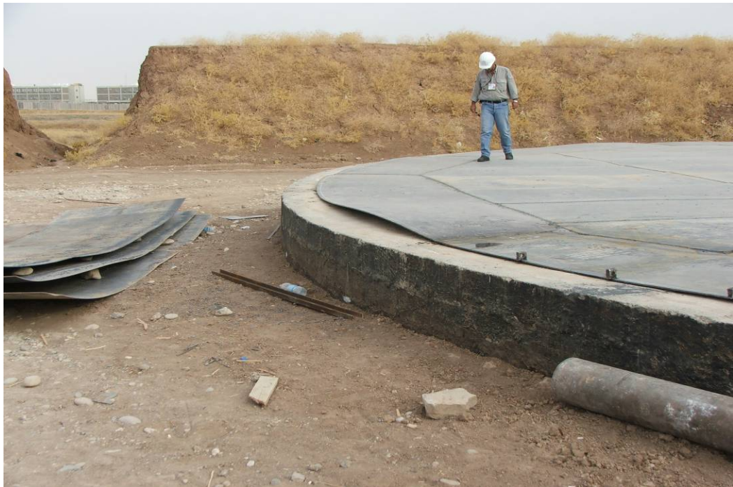
Site Photo 4. Steel floor placed on concrete foundation
