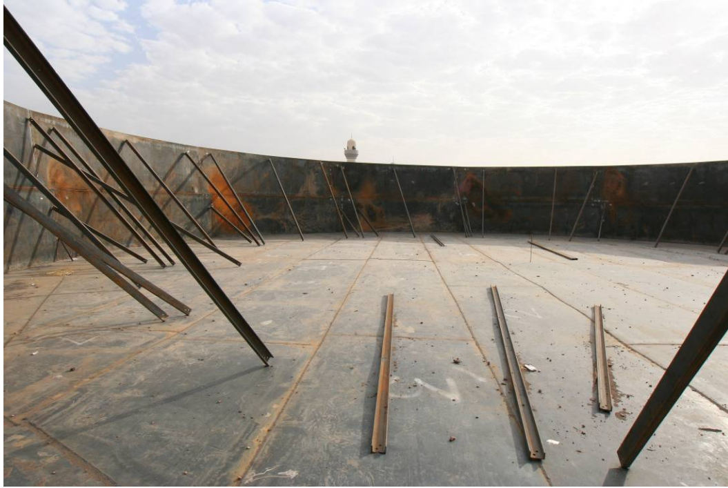
Site Photo 17. Inner tank bracing supports the attached steel shell plates.
