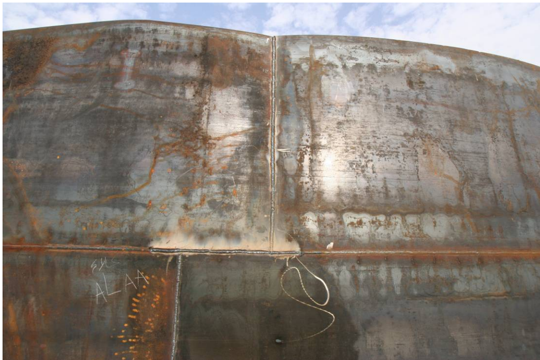
Site Photo 24. Completed second run on a vertical weld of a shell plate.
