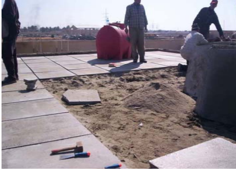
Site Photo 8. Contractor repairing the guard house roof after being notified by SIGIR (From Weston photo log)
